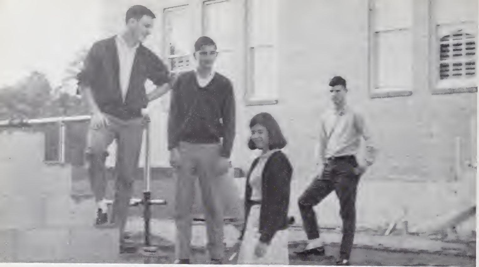
Officers of the Sophomore class inspect the framework of the new buildings on campus. They anticipate the many activities that will be conducted in these buildings. The officers are John Walston, Treasurer; Alan Strickland, President; Debrs Thorne, Secretary; and Danny Cole, Vice-President.
