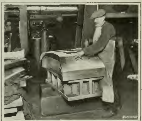
Fig. 2. Hand Filing a Die after removing it from Die-sinking Machine
