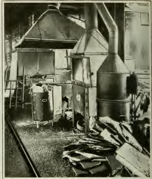
Fig. 8. Furnaces used for the Recovery of Solder from Sheet Metal
