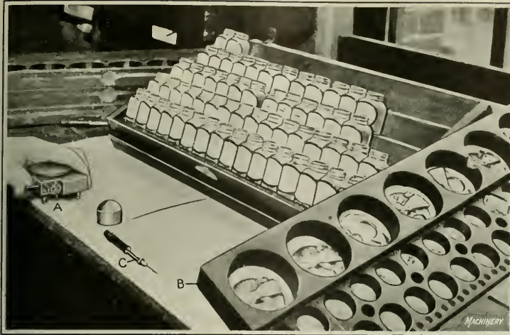
Fig. 2. Equipment used for inspecting Watch Staff Pivots and Jewels
