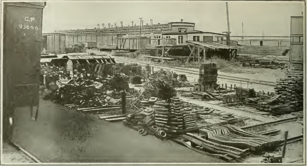
Fig. 1. Partial View of Storage Space in which Usable Materials are kept in Bins carrying their Part Numbers
