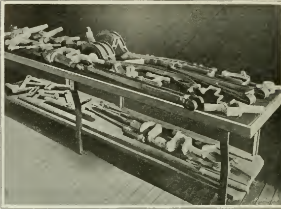
Fig. 1. Examples of Drop-forgings, showing Variety of Size and Design
