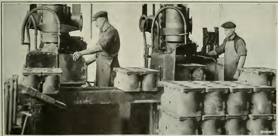
Fig. 4. Surface-grinding Operation on Cylinder Castings
