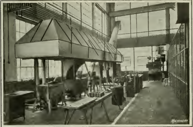
Fig. 8. Heat-treating Department—Note Provision of Overhead Hood for carrying off Fumes and Smoke
