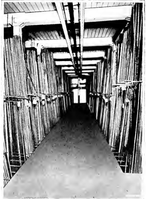
Fig. 3. Aisle in Storage House where Different Sizes of Bar Stock are stored
