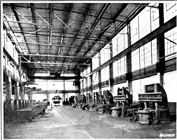
Fig. 1. View in Front Head-house used as Erecting Floor
