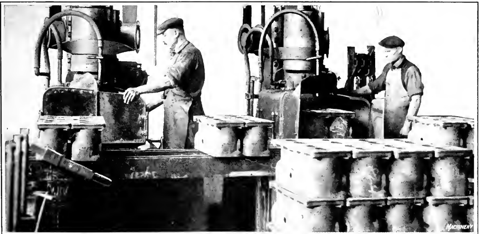
Fig. 4. Surface-grinding Operation on Cylinder Castings
