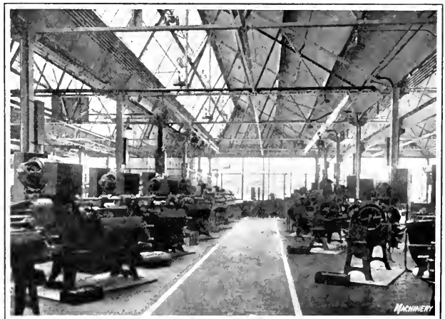
Fig. 6. Aisle in the Automatic Screw Machine Department, showing Individual Motor Drive
