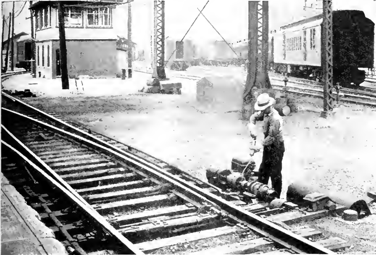
With Alemite, all the operator has to do is to attach the flexible hose to any fitting—give the compressor handle a turn or two—and clean lubricant shoots into the bearing under 500 pounds' pressure
