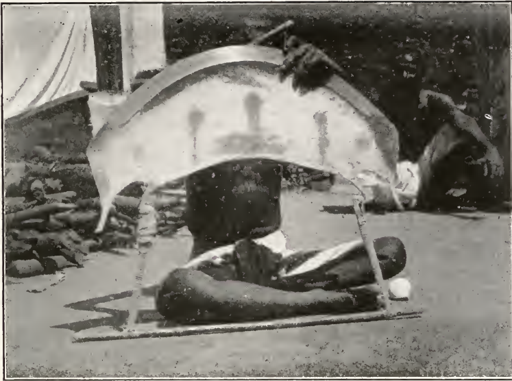
FIG. 1.—SHARPENING A CHANK SAW, DACCA.
