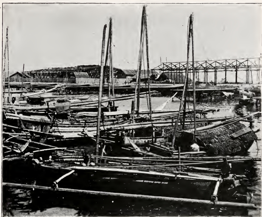
FIG. XVIII.—DOUBLE OUTRIGGER WITH SUB-DIRECT ATTACHMENT, MACASSAR.
