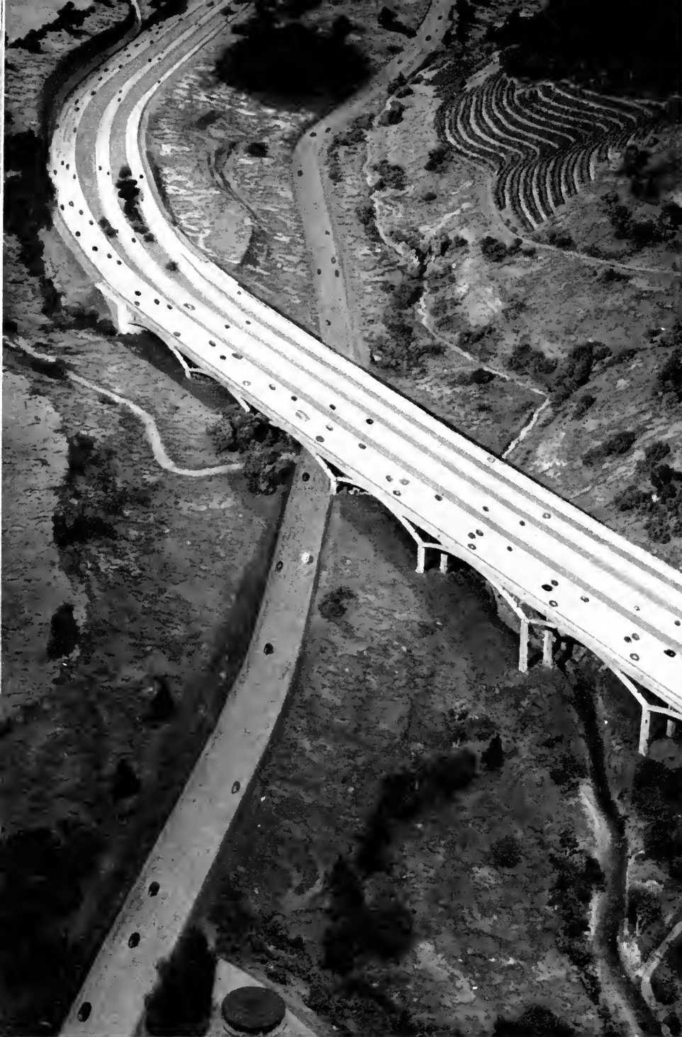
MOTORWAYS FOR INCREASED DISTRIBUTION
