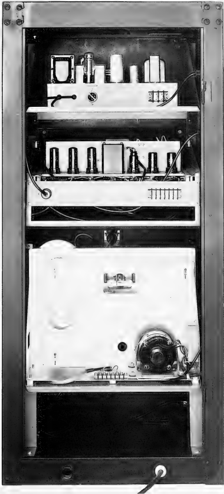
FIG. 7 - Rack Two, Rear View
