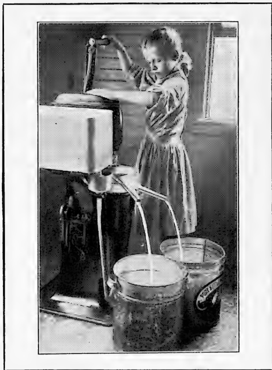
Running the separator.
