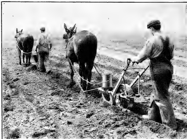
A Fertilizer Distributor and Planter. The fertilizer is applied first and then the planter puts down the seed. Good seed and fertilizer will increase your yields per acre.
