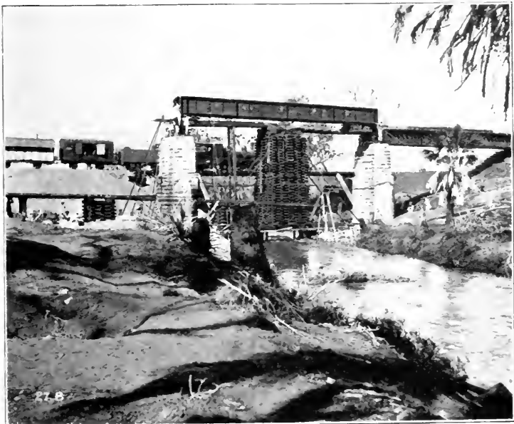
"AND FINALLY LOWERED GENTLY INTO POSITION."
