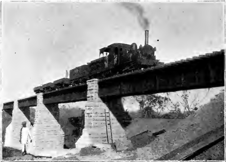
"VERY SOON I HAD THE SATISFACTION OF SEEING THE FIRST TRAIN CROSS THE FINISHED WORK."
