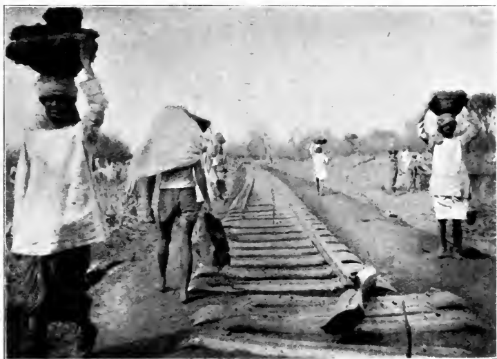
“ANOTHER GANG DROPS THE RAILS IN THEIR PLACES.”
