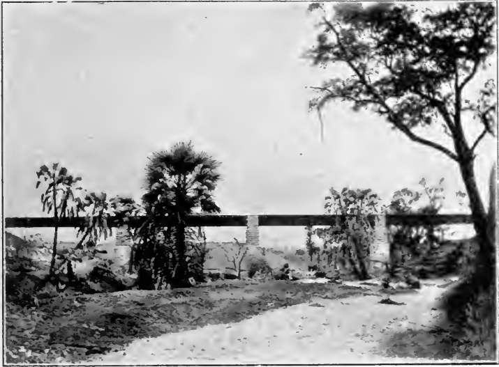
FIG. COMPLETED TSAVO BRIDGE.
