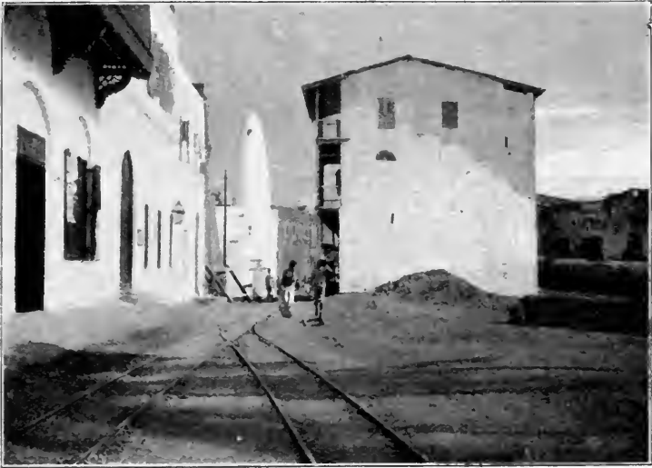
VASCO DA GAMA STREET AND PILLAR.
