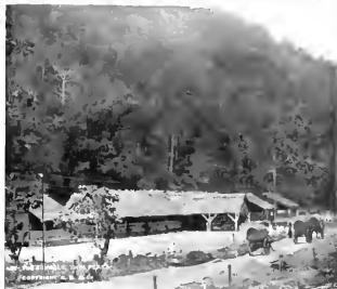
Fig. 1. The main building at the station.
