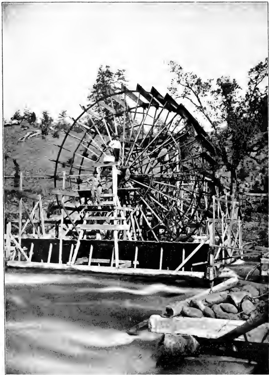
CURRENT-WHEEL FOR PUMPING WATER AT BAIRD, CALIFORNIA.
