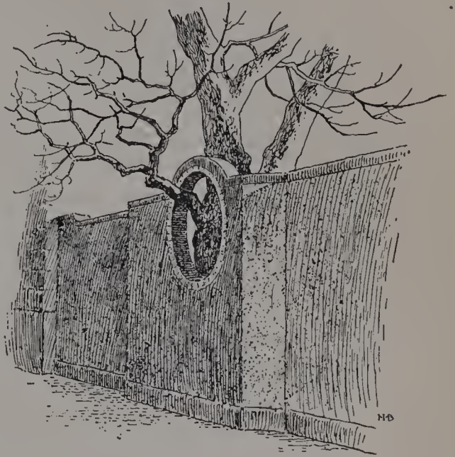
165. Accommodating a wall to a valuable tree.
