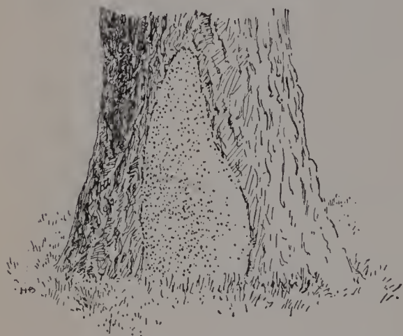
160. A cement-filled cavity at the base of a tree.
