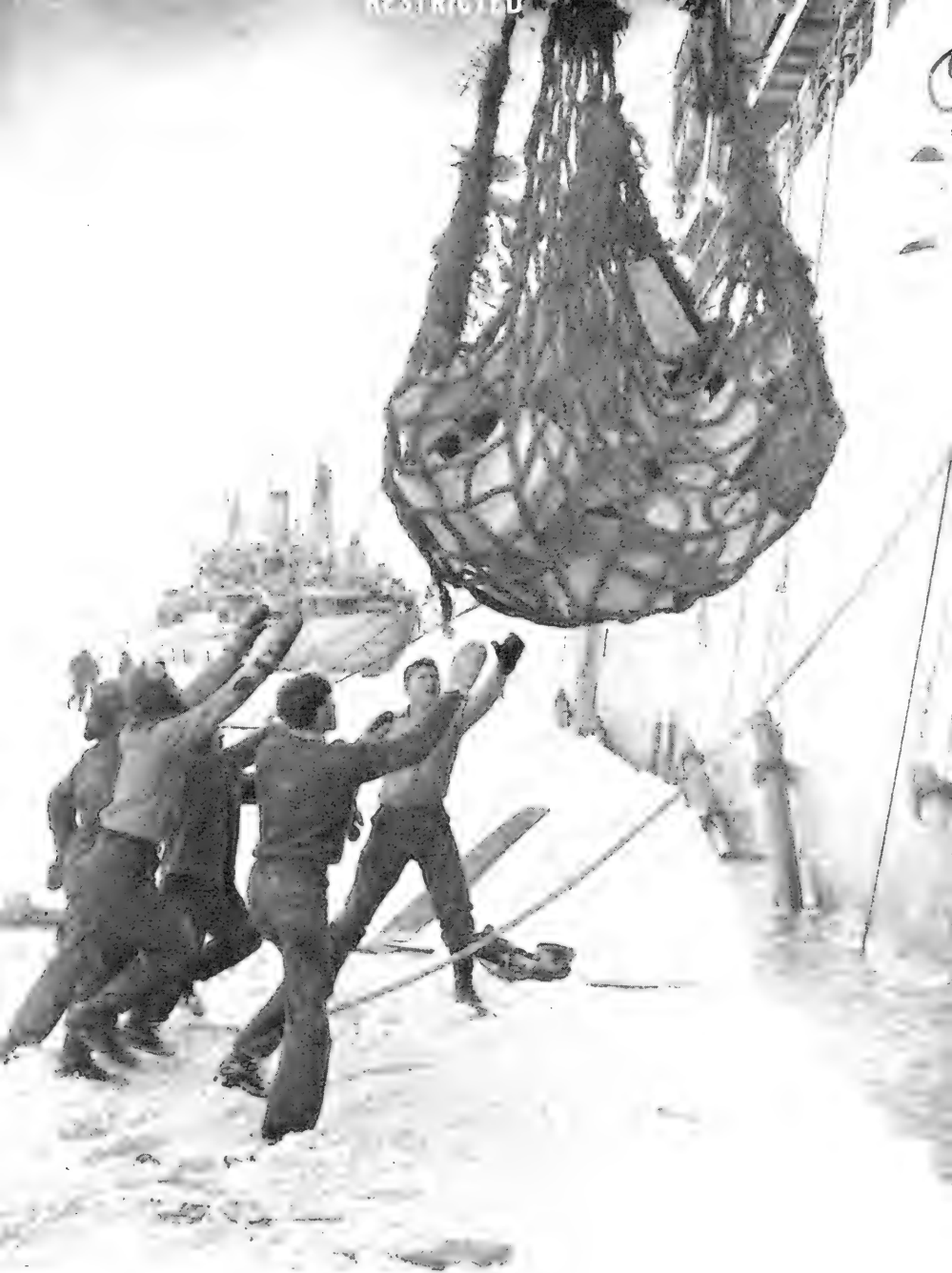
Figure 15.—Unloading cargo from U. S. S. Yancey (U. S. S. Merrick in background). Lengths of telegraph poles hung vertically over side of ship are used as fenders.
