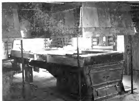
Figure 73.—A canopy-type hood removes steam more efficiently than do louvers. However, large volumes of air are required to sweep the steam into and up through the hood and the result is a cold, drafty building.
