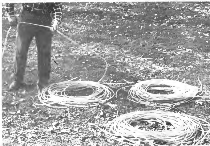
Figure 55.—Coiling lateral lines for ease of handling.
