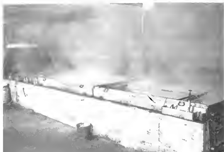
Figure 72.—Evaporator house with opening in the roof for venting the steam results in a steam-filled building.
