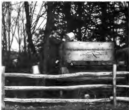
PN-4729 Figure 33.—Collecting tank mounted on a truck body. This type of assembly does not require special rigs, but an additional man is needed to empty the pails into the tank.
