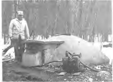
Figure 67.—A large underground concrete storage tank of silo-type construction.
