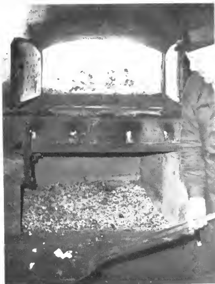
Figure 127.—Where coal is inexpensive, high-pressure steam boilers may be used to evaporate sap to sirup.
