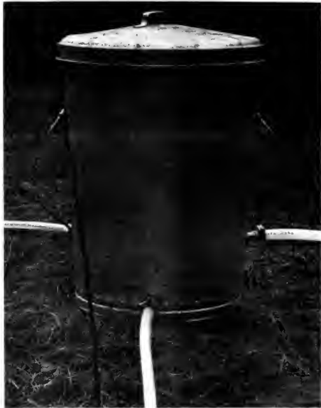
Figure 45.—Junction of several main lines with surge tank and vent.
