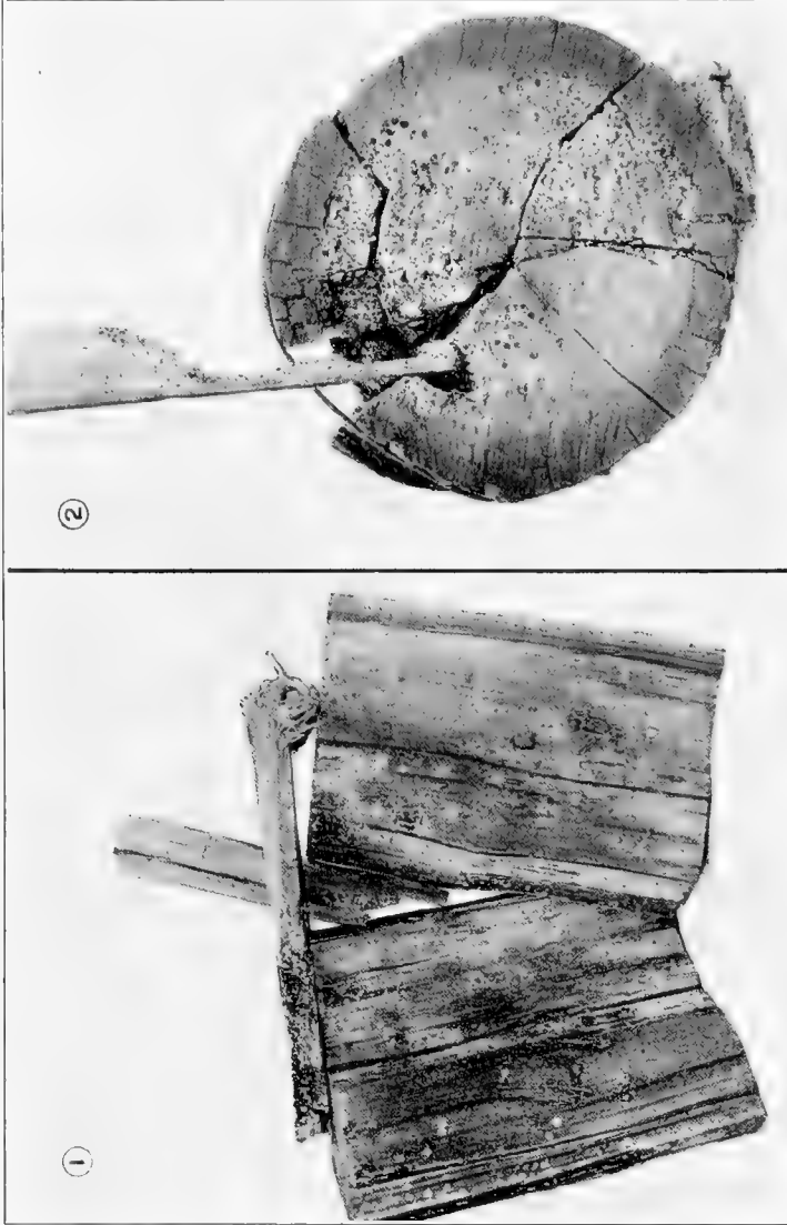
Fig. 25. (1) Vertical section, and (2) cross-section through portion of a perfectly treated pile which was split and broomed during driving. Ixodes entered splits and worked through untreated heartwood to the creosoted outer shell, which was attacked in a few spots as shown by smaller pieces.
