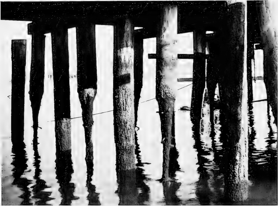
Fig. 13. Untreated Douglas fir piling in Oakland Estuary, destroyed by Limnoria . Good piles shown are replacements. (Moore Shipbuilding Co. Photo.)
