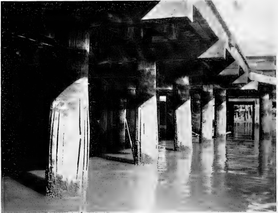
Fig. 56. Piling treated by Moran process, exposed 2 years at Georgia St. Wharf, Vallejo. Note bulging and broken battens. (S. P. Co. Photo.)
