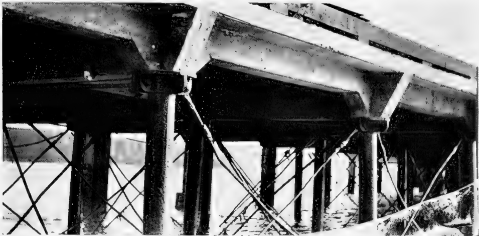
Fig. 58. Iron piling at Fort Baker.
