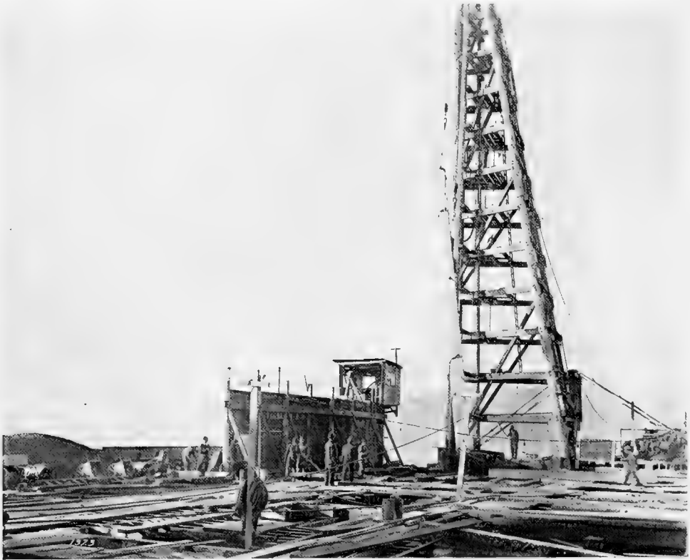
Fig. 23. Handling 100-ft. concrete piles during pier construction.
