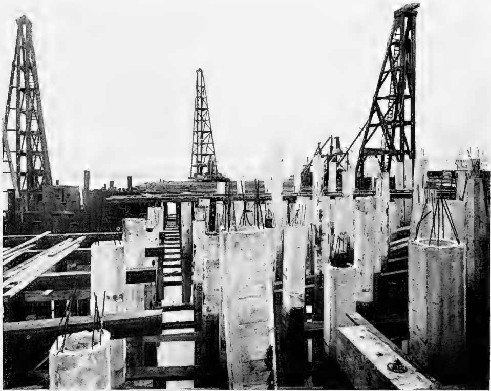
Fig. 47. Pre-cast concrete jackets in place over piles. Alaska Packers' Assn., Alameda.
