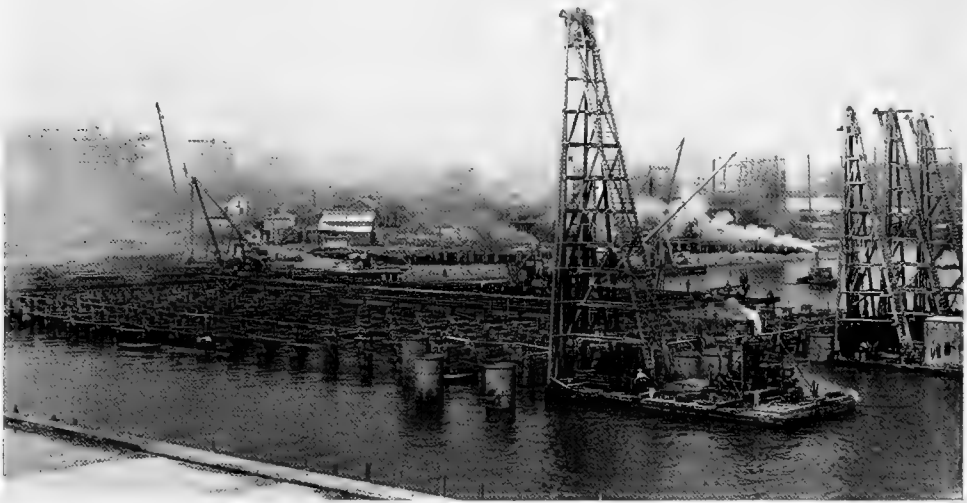
Fig. 10. Driving cylindrical cofferdam forms, pier 36, August, 1909.
