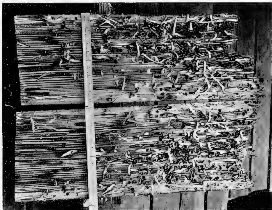
Fig. 90. Split section of pile shown in fig. 89.
