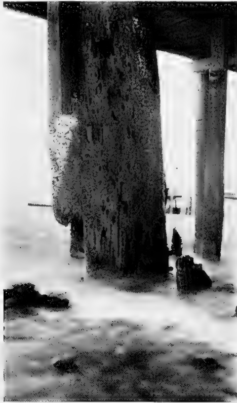
Fig. 139. Pile at China Camp, on the west shore of San Pablo Bay, attacked by Sphaeroma pentodon between tide levels.
