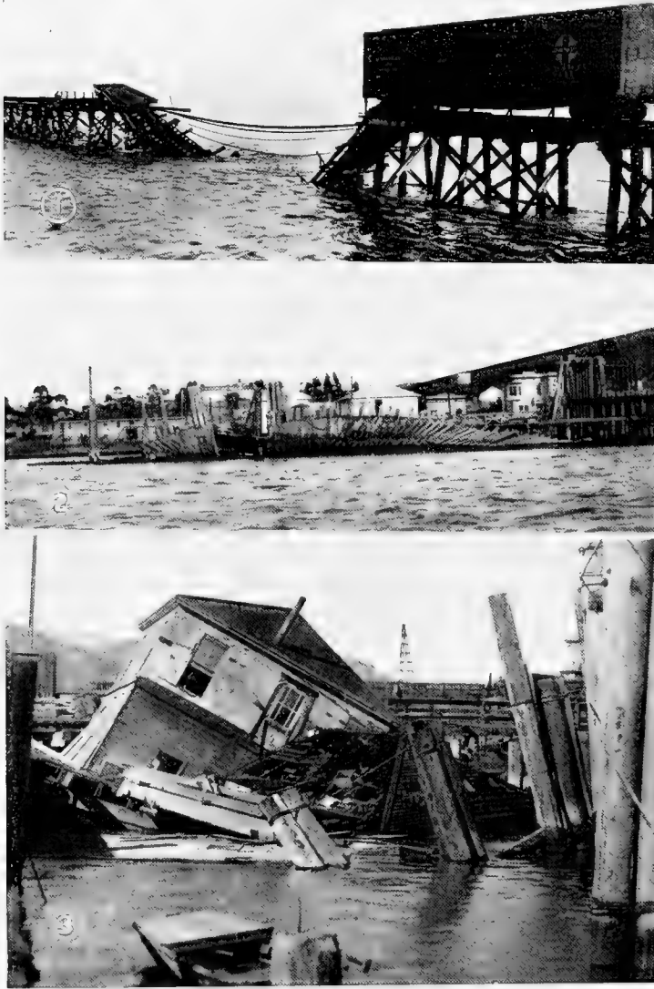
Fig. 1. Dock failures in Carquinez Strait.
