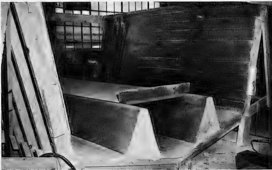
Fig. 4-13. Polyurethane foamed in place cores for main longitudinals of 36' LCVP test section (Courtesy Budd Company)
