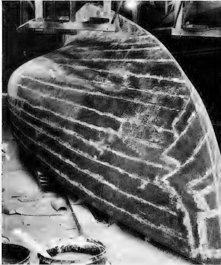
Fig. 4-17. Fiberglass hull of a 40' ketch molded on a male form (Courtesy Jean Filloux)
