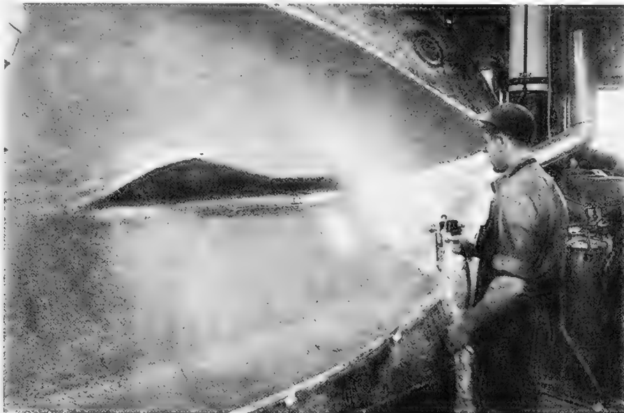
Fig. 4-16. Molding of hull of sailboat in female mold. Resin mix being sprayed on reinforcement (Courtesy American Carbide Corporation)
