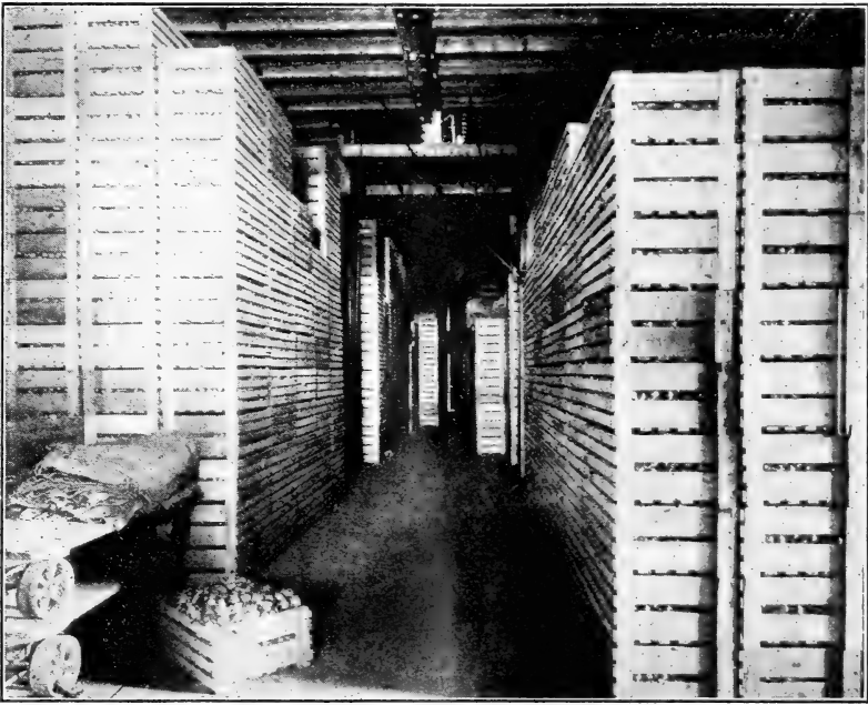
FIG. 12.—Interior of onion-storage house
