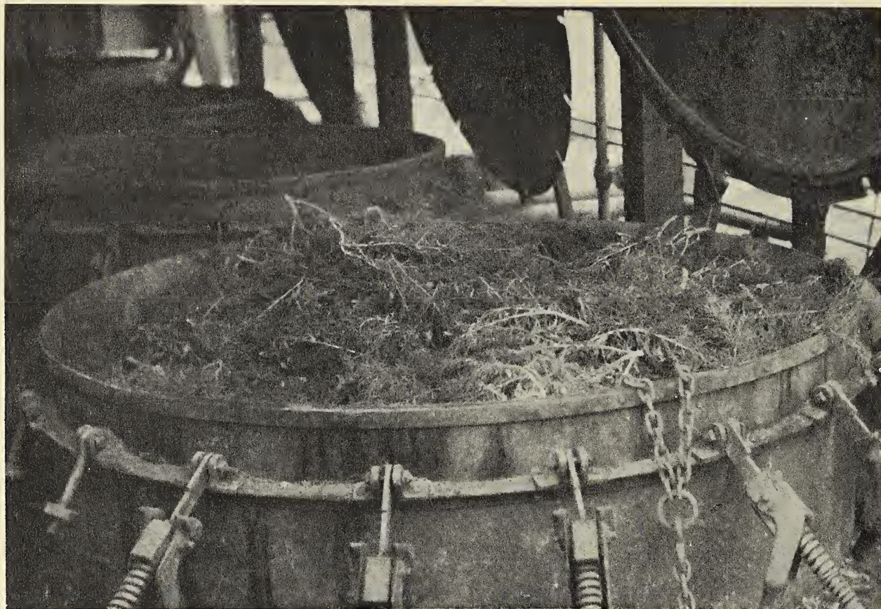
Fig. 2 Wormseed in distillation kettle
