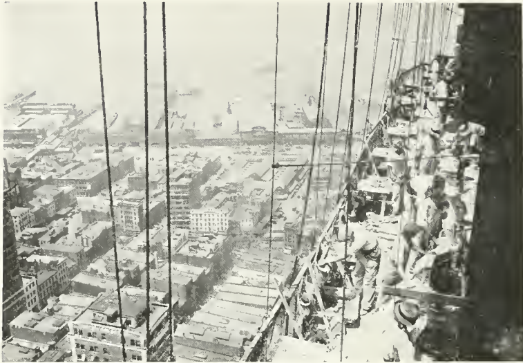
SUSPENDED PLATFORMS—PATENT SCAFFOLDING CO.
