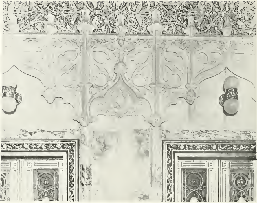
PLASTERING—H. W. MILLER, Inc.
