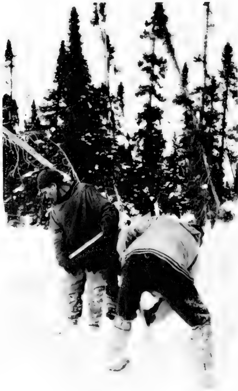
FIG. 6. Loose surface snow being scraped off with wooden shovels prior to the construction of a ridgepole lodge (neg. no. 61703).
