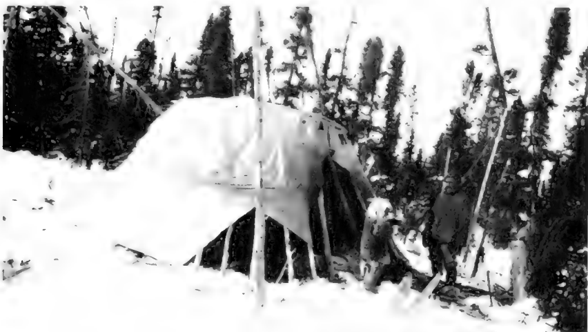
FIG. 18. Completing the covering of the lodge frame (neg. no. 69598).
