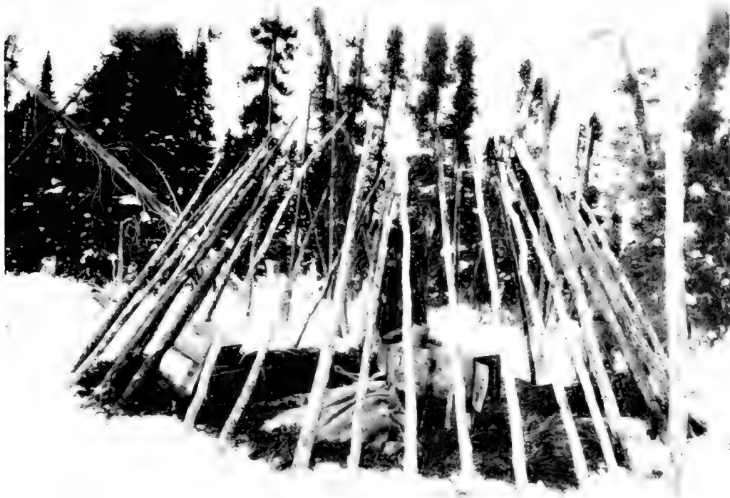
FIG. 13. Wall poles and spruce bough floor in place (neg. no. 61660).
