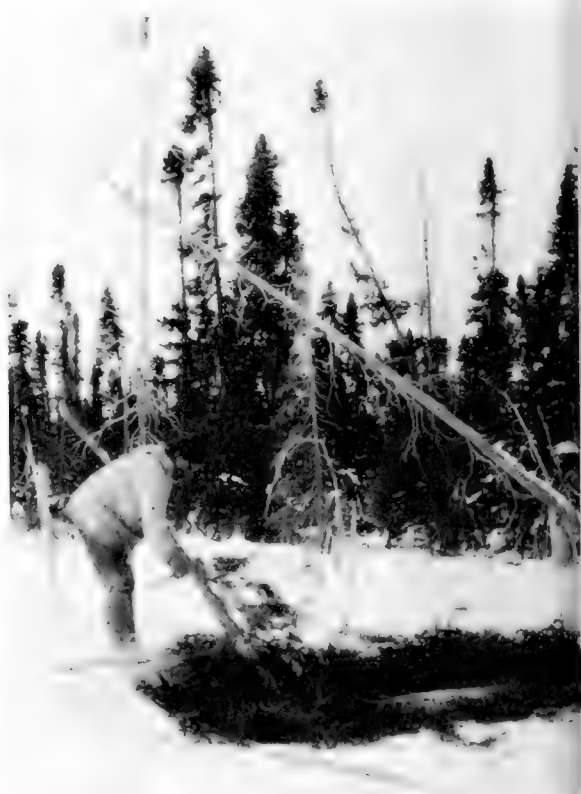
FIG. 7. Joe Rich stripping boughs from spruce poles to be used in the construction of the lodge (neg. no. 61556).
