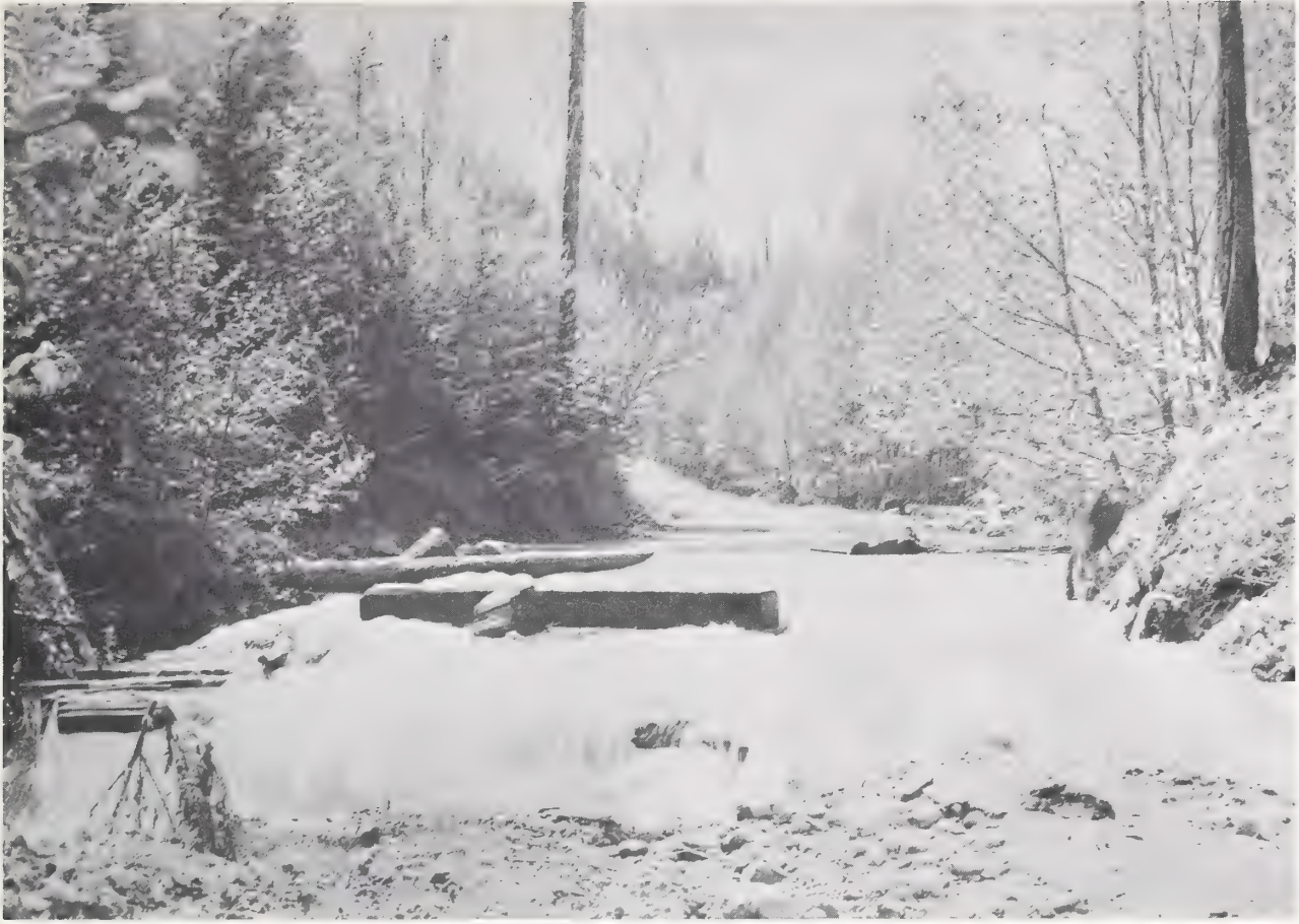
A raging mountain stream overflows a bridge.
