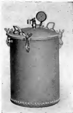
FIG. 121. Pressure canner showing pet cock.
