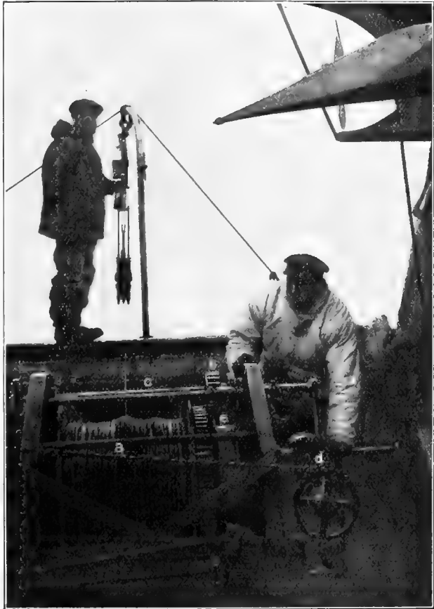
Fig. 2. Winch for soundings and hydrographical work; C. B. Thostrup phot.
