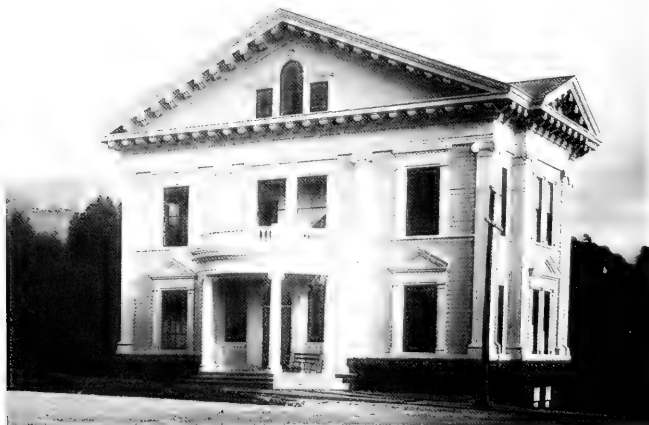
FIGURE 21. Botany Building, University of California, Berkeley (circa 1898). Courtesy University Herbarium Archives, University of California, Berkeley.
