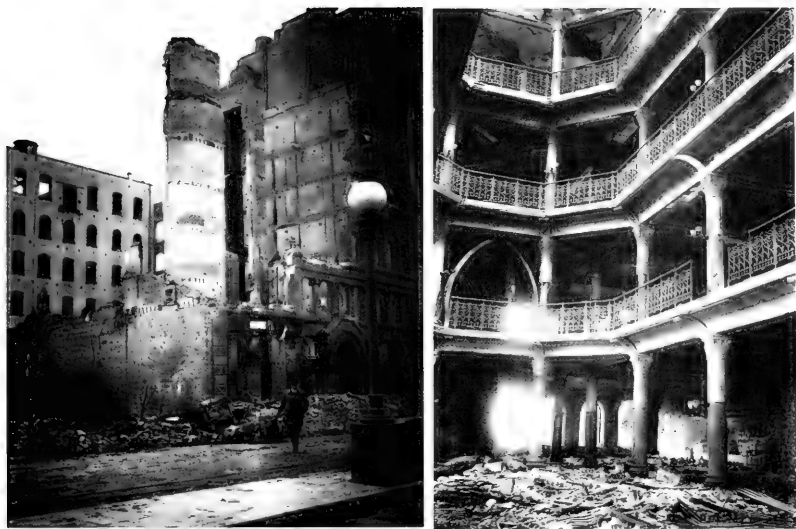
FIGURES 27–28. (27) The remains of the California Academy of Sciences following the devastating earthquake and fire of 18–19 April, 1906. The elevator shaft alone remains standing of the Market Street building; the building immediately behind and to the left was the Academy's museum building. (28) The interior of the Academy's museum building following the devastating earthquake and fire of 18–19 April, 1906. California Academy of Sciences Archives.
