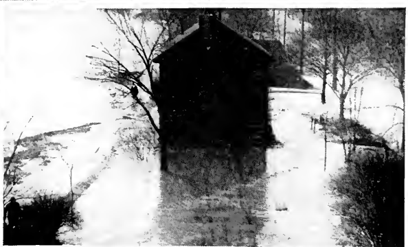
"OLD LOG CABIN" OVER 100 YEARS OLD, WITHSTOOD DAYTON, O., FLOOD, 3 - 26 - 13
