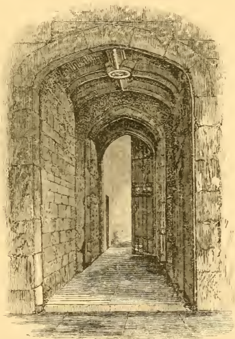
SIDE PASSAGE, BYWARD TOWER.
