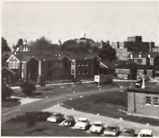
Broughton Hospital, Morganton, N. C.
