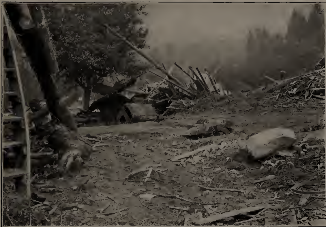
(A) FLOOD DAMAGES TO MINING SETTLEMENT, NORWOOD, W. VA., 1901.
