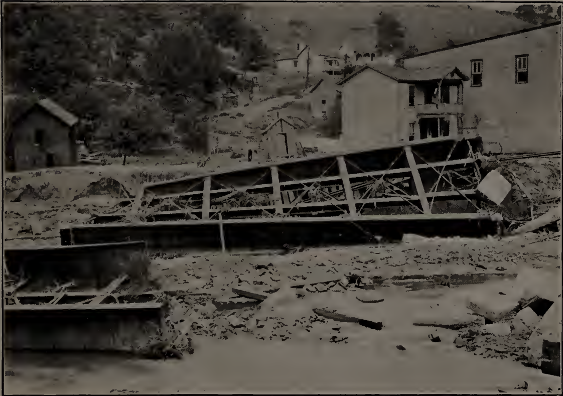
(A) FLOOD DAMAGES ON ELKHORN CREEK, IN WEST VIRGINIA, JUNE, 1901.
