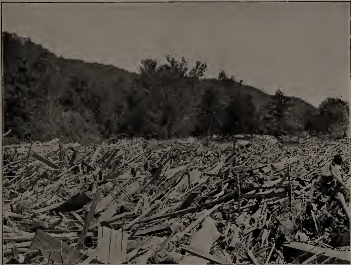
(B) DÉBRIS FROM FLOODS ON NOLICHUCKY RIVER, EAST TENNESSEE, MAY 21, 1901.
