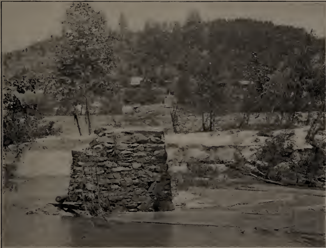
(A) HIGHWAY BRIDGE WASHED AWAY BY FLOODS. (See pp. 32, 130.)
