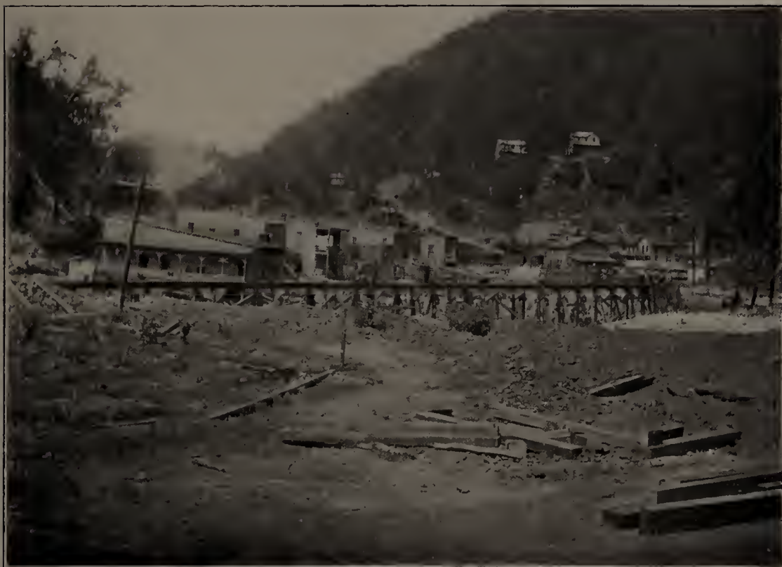
(B) FLOOD DAMAGES TO RAILROAD AND MINING SETTLEMENT, KEYSTONE, W. VA., 1901.
