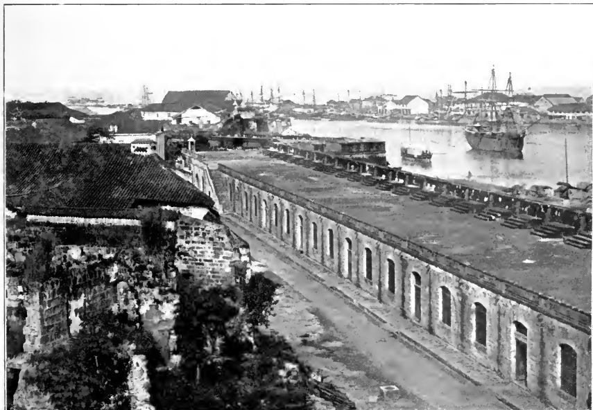
RUINS OF CUSTOM HOUSE, EFFECT OF EARTHQUAKE, 1863.
