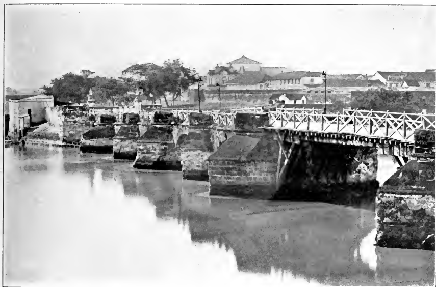
STONE BRIDGE OVER RIVER PASIG, PARTLY DESTROYED BY AN EARTHQUAKE, 1863.
