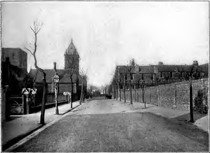
OLD CHURCH OF ST. AUGUSTIN, NOW CHAPTER HOUSE—OBSERVATORY, ABBEY OF ST. AUGUSTIN.
