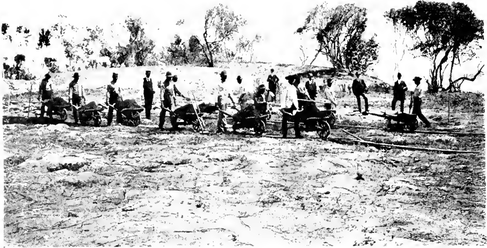
Starting Miami. Breaking Ground for Royal Palm Hotel, March 15, 1936
