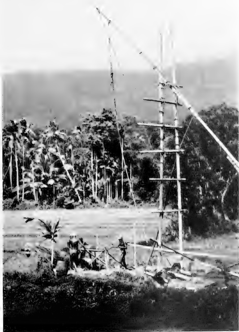
Singhalese sinking a shaft for sapphires, Palmadulla, Ceylon. (Photo by F. D. Adams)
