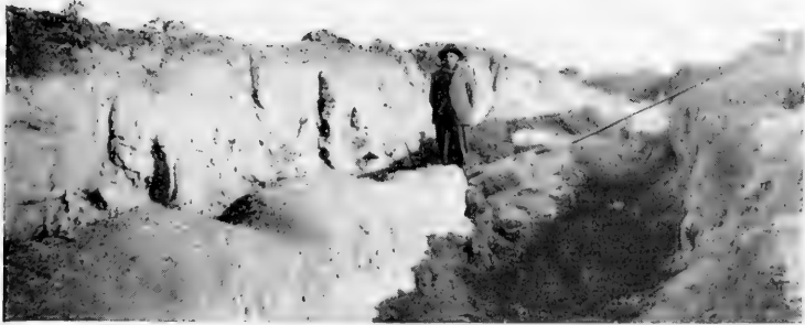
Trenches in decomposed diamond-bearing peridotite, Arkansas mine, Pike County, Arkansas. (After Miser and Ross, U. S. Geological Survey)
