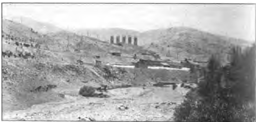
Photo No. 6. Mammoth Smelter; bag house in center.
