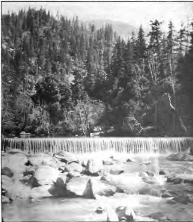
Photo No. 4.—Dam—Forks of Salmon River Mining Company.
