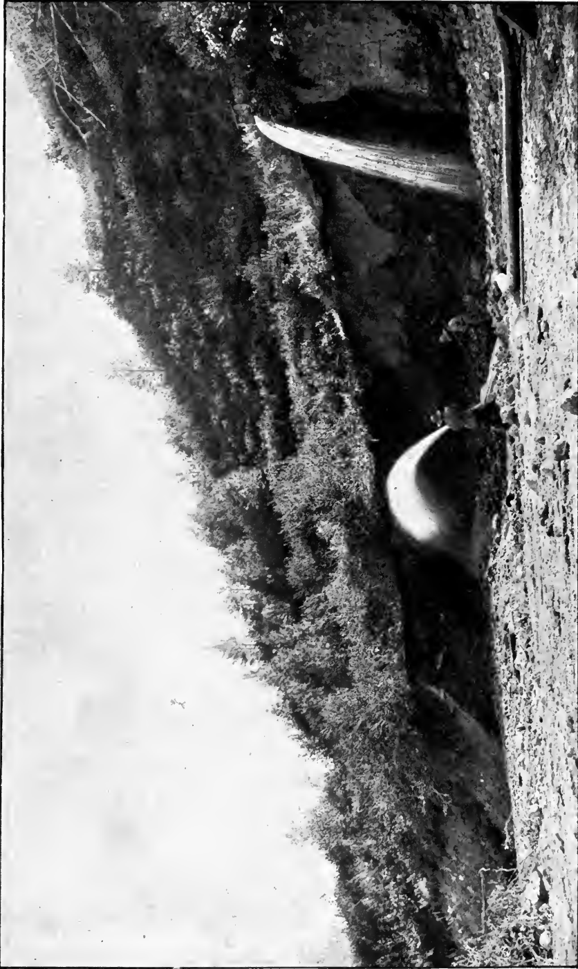
WORKING BENCH GRAVEL BY THE HYDRAULIC PROCESS AT IDAHO CITY.
