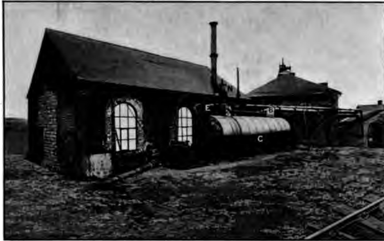
FIG. 11.—VIEW OF PLANT.
