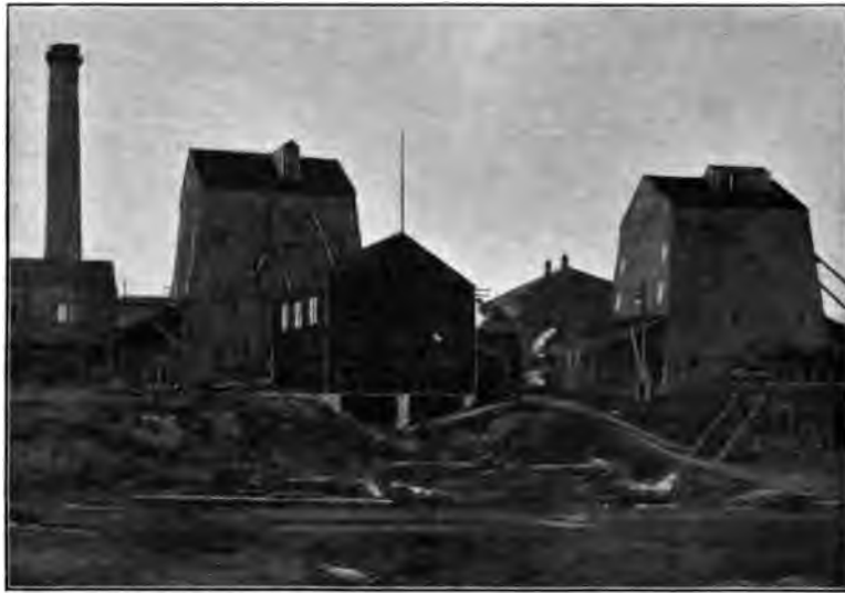
FIG. 34. — EAST SIDE OF SINKING-SHEDS AND FREEZING-HOUSE.
