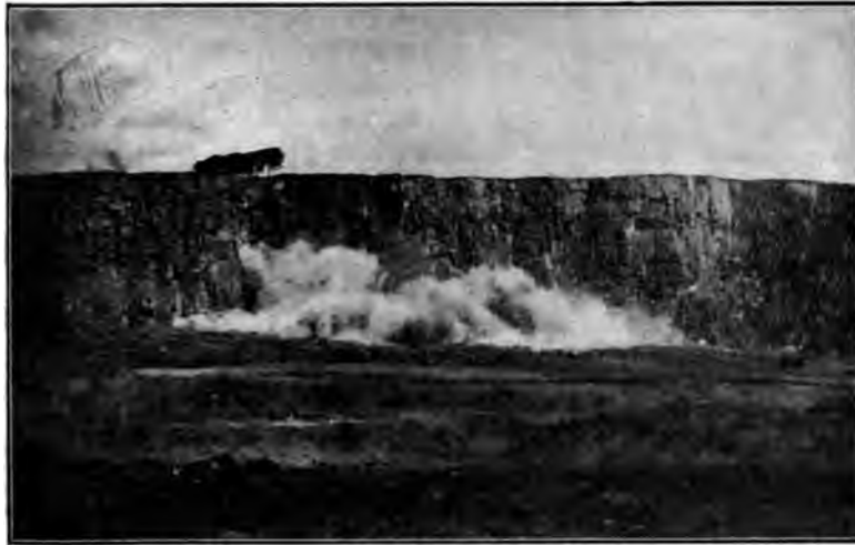
FIG. 1.—BLAST DISLODGING 30,000 TONS OF CARBONIFEROUS LIMESTONE, a to b, IN CAULDON LOW QUARRIES.
