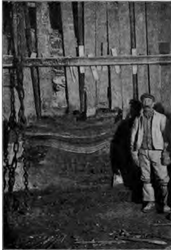
FIG. 39.—DRIFT BETWEEN THE CASTLEREAGH AND THERESA SHAFTS, AS FOUND IN THE CASTLEREAGH SHAFT.
