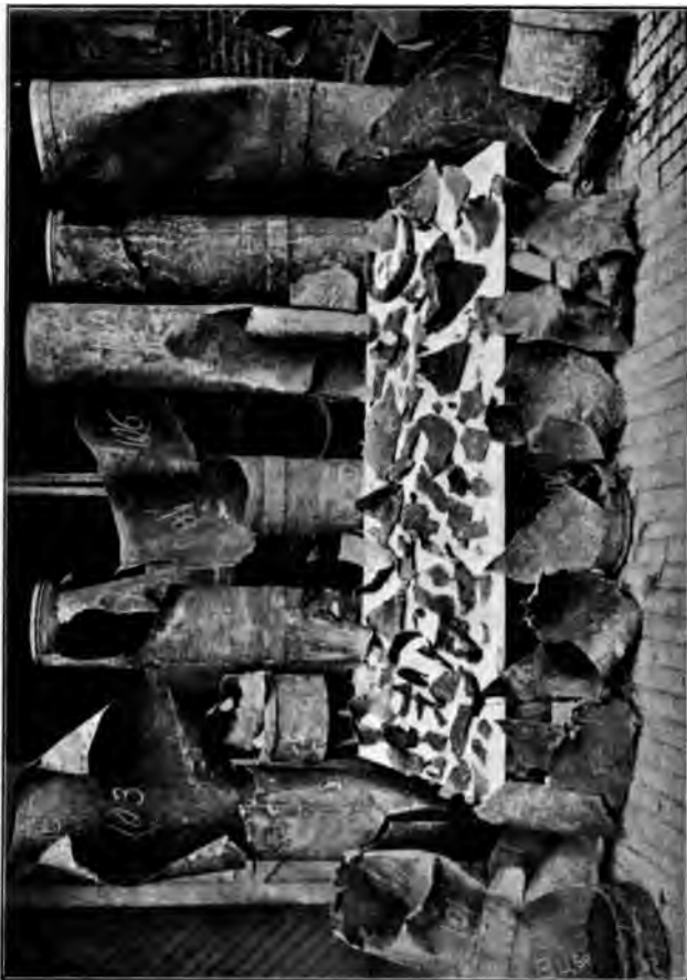
FIG. 22. — BROKEN AIR-PIPES FROM LECŒUVRE HEADING.
