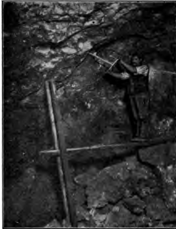
FIG. 10.—MAN BORING A SHOT-HOLE IN FAULD MINE.
