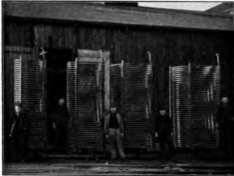
FIG. 37.—SPIRAL TUBES FOR COOLING-CONDENSERS AND REFRIGERATION-TANKS.
