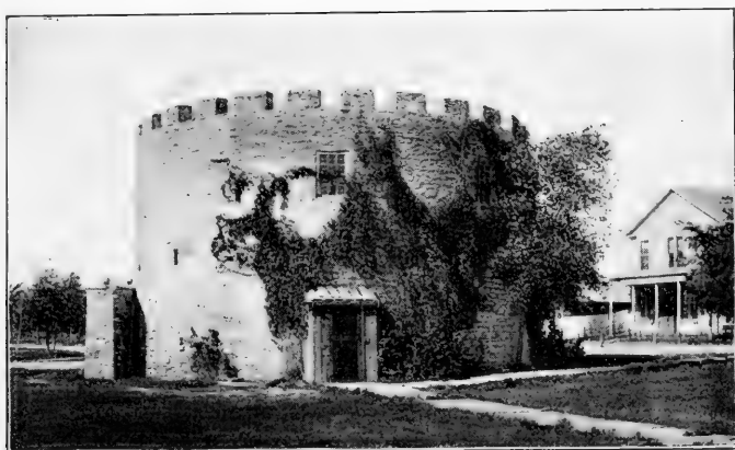
FIG. 217.—The Virginia creeper on the walls of the old round tower, Fort Snelling. This plant does not turn towards the sun, but clings to the shaded wall. After photograph by Williams.
