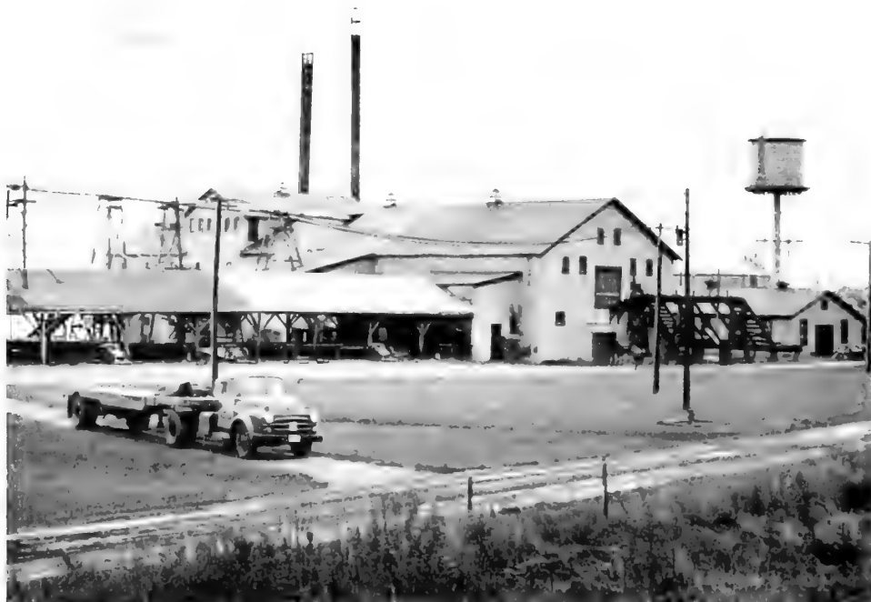
FIGURE 25.—One of the largest mills in the State is the Red Lake Indian Mills at Redby. It is an 8-foot band mill with a 6-foot horizontal resaw, 66-inch double edger and trimmer. Auxiliary units consist of a planing mill, lath mill, fishbox factory, and electric-power generator for the local community. The mill organization markets all the lumber, boxes, cedar posts, poles, and pulpwood produced on the Red Lake reservation.
