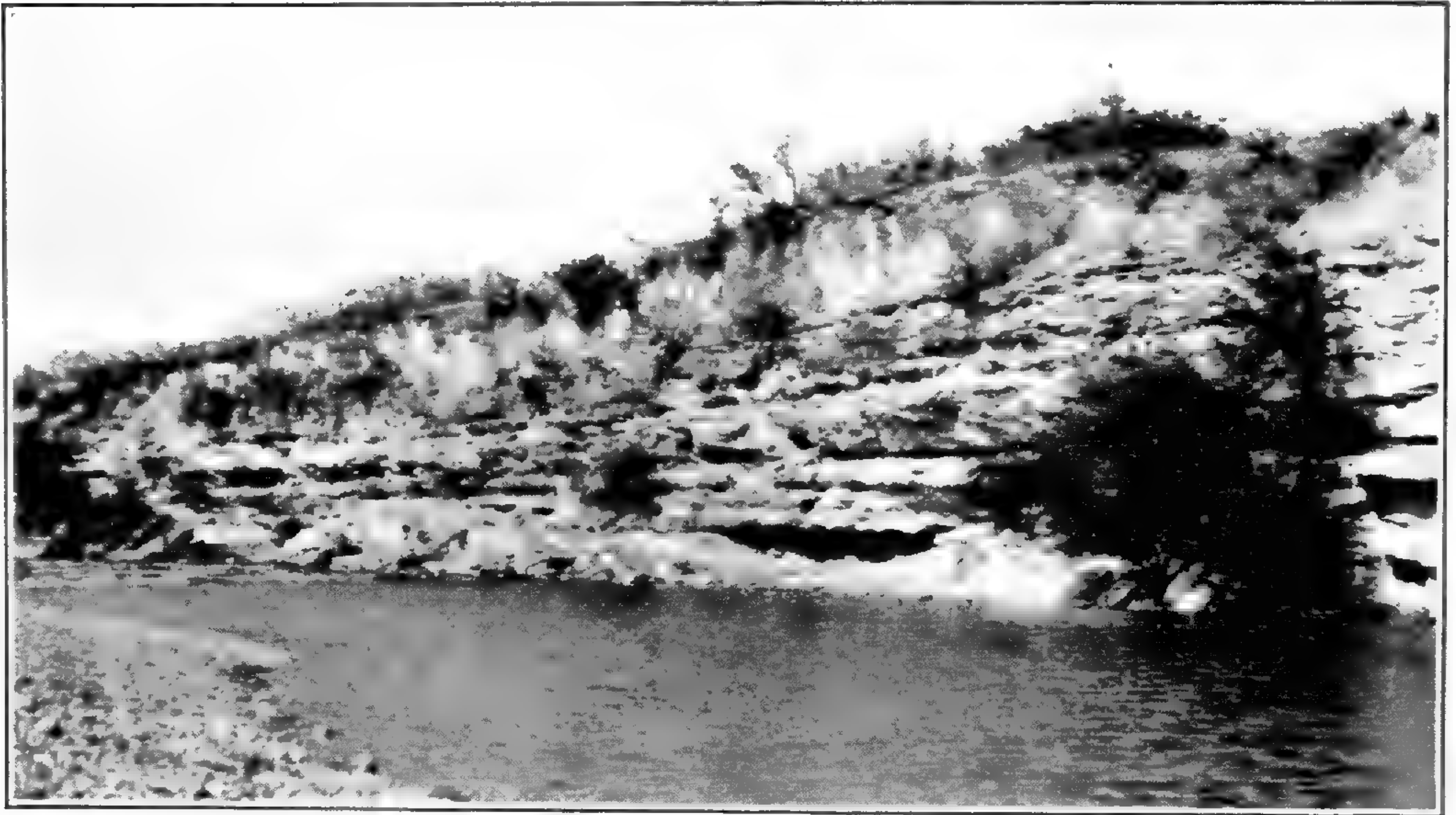
A. ANACACHO LIMESTONE AT KING'S WATER HOLE, 3 MILES NORTH OF HONDO, TEX.
