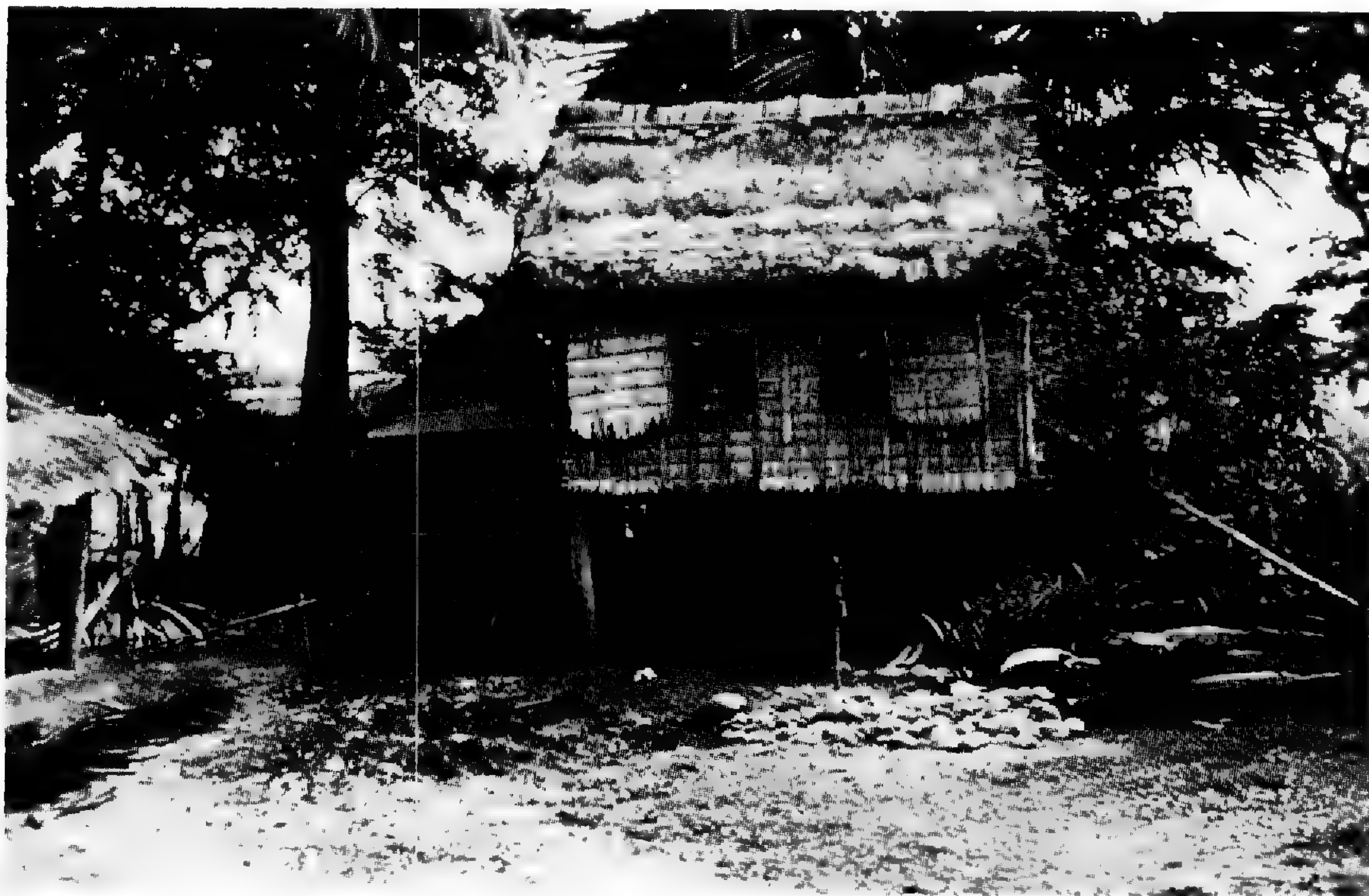
A typical hut constructed mostly of bamboo and palm leaves, in the Manila Plain.
