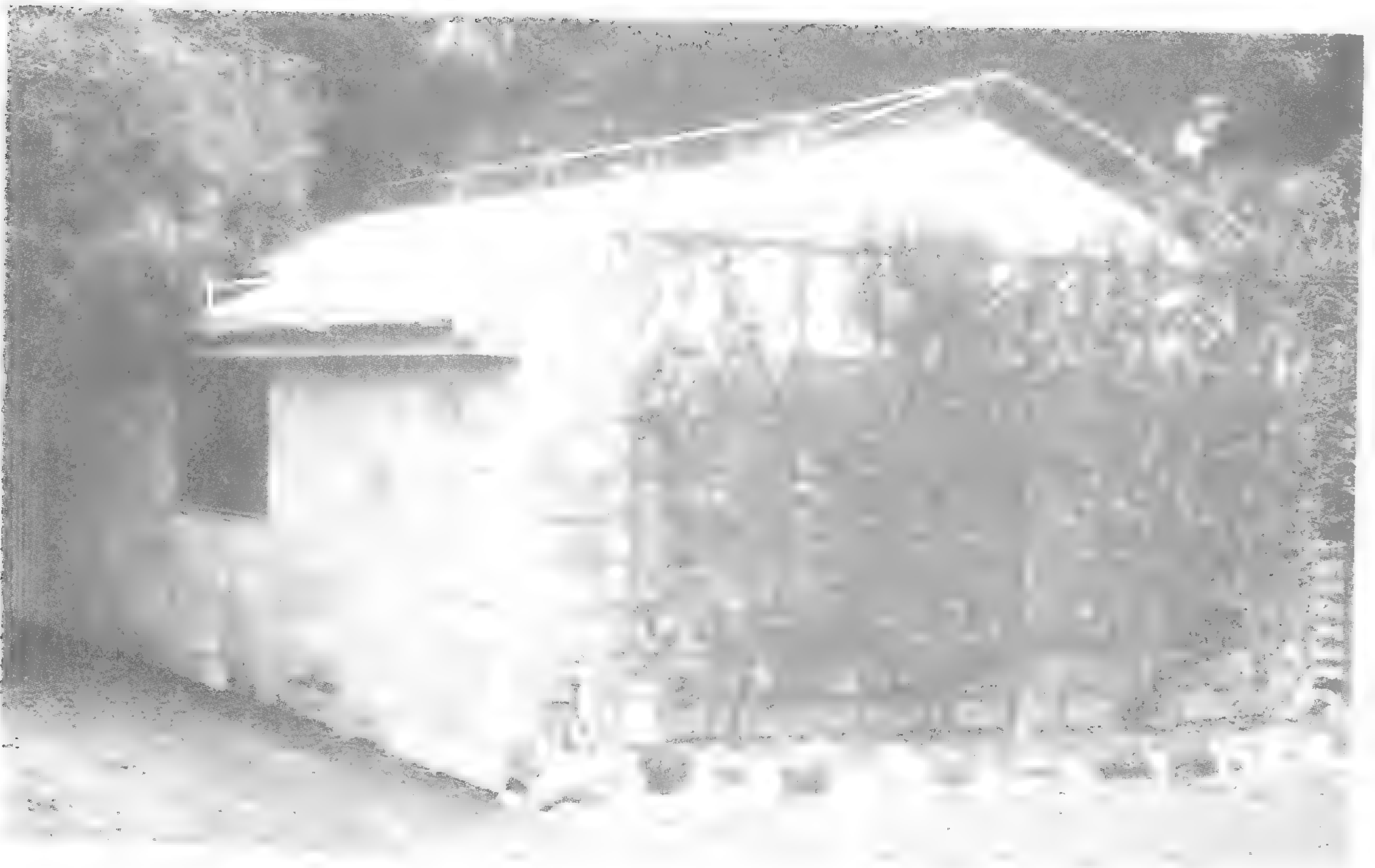
Fig. 4 The filmy-fern house showing the double-glazed window and outer door. The pipe frame mounted above the roof is used in summer for shade cloth, although it is not being used this year
