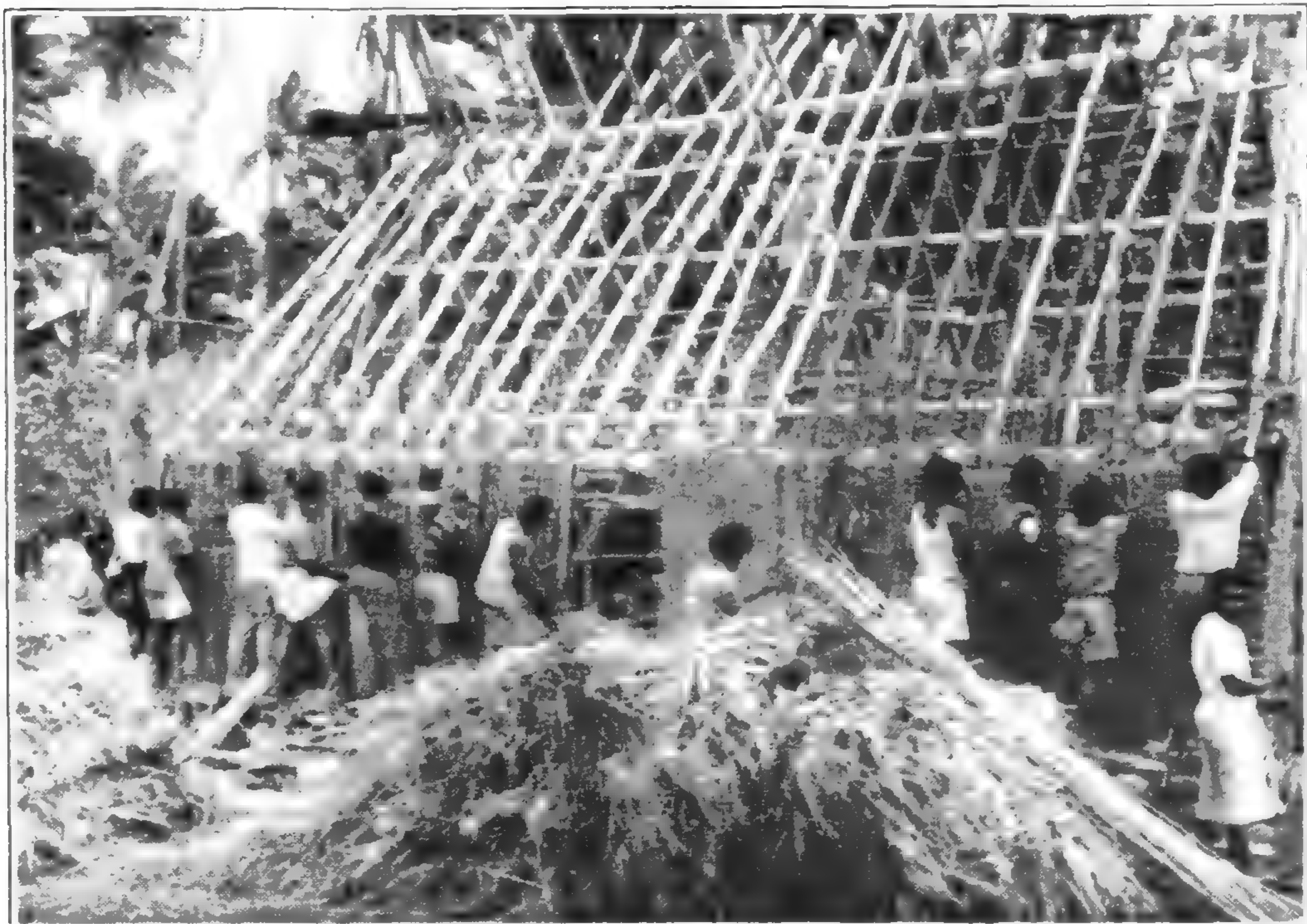
A. CONSTRUCTION OF HOUSE, SHOWING CADEX OF CYATHEA LUNULATA ATTACHED TO END OF RIDGE-POLE.
