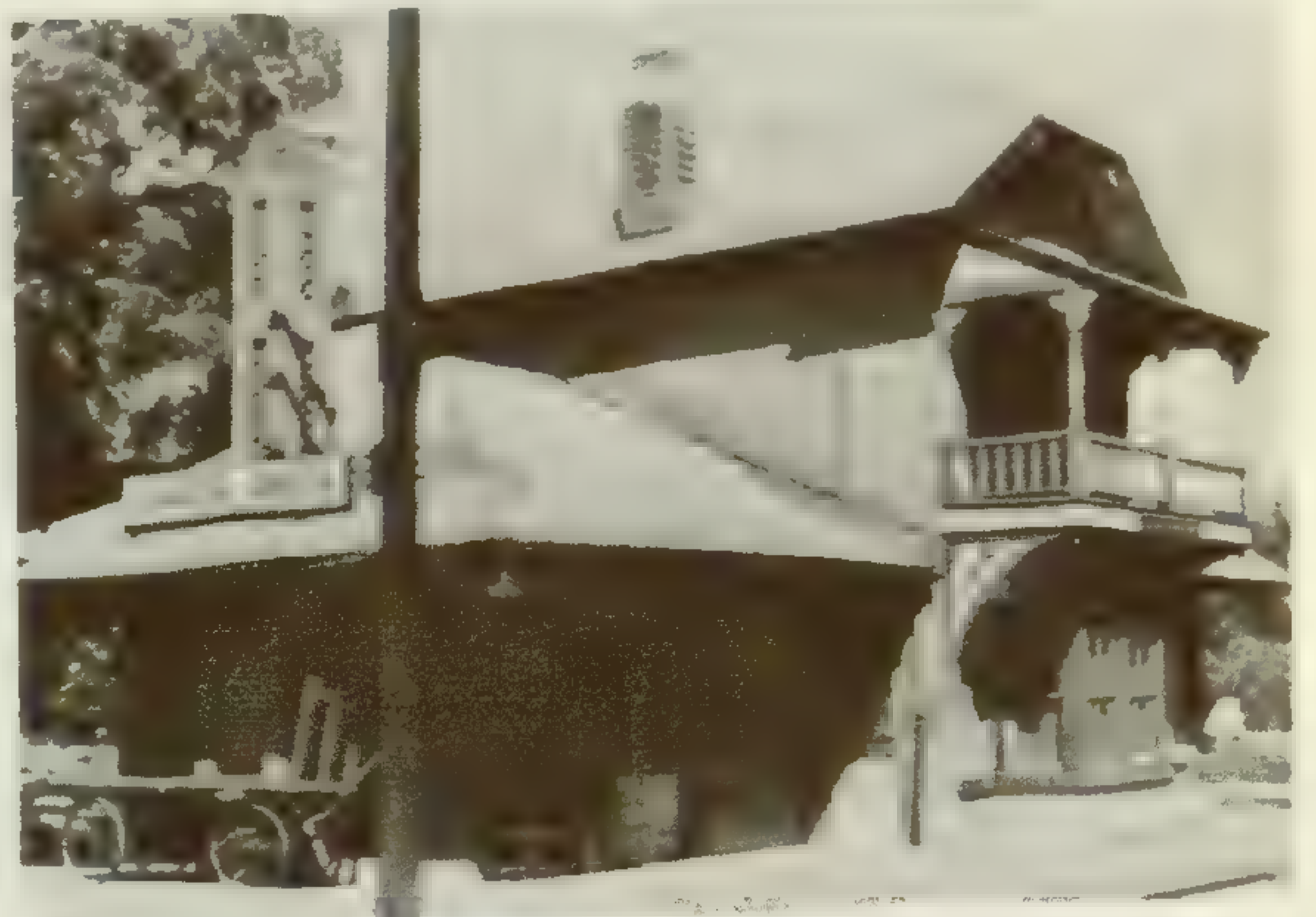
This is the way the depot looked in May, 1940, when it was closed for the last time.
