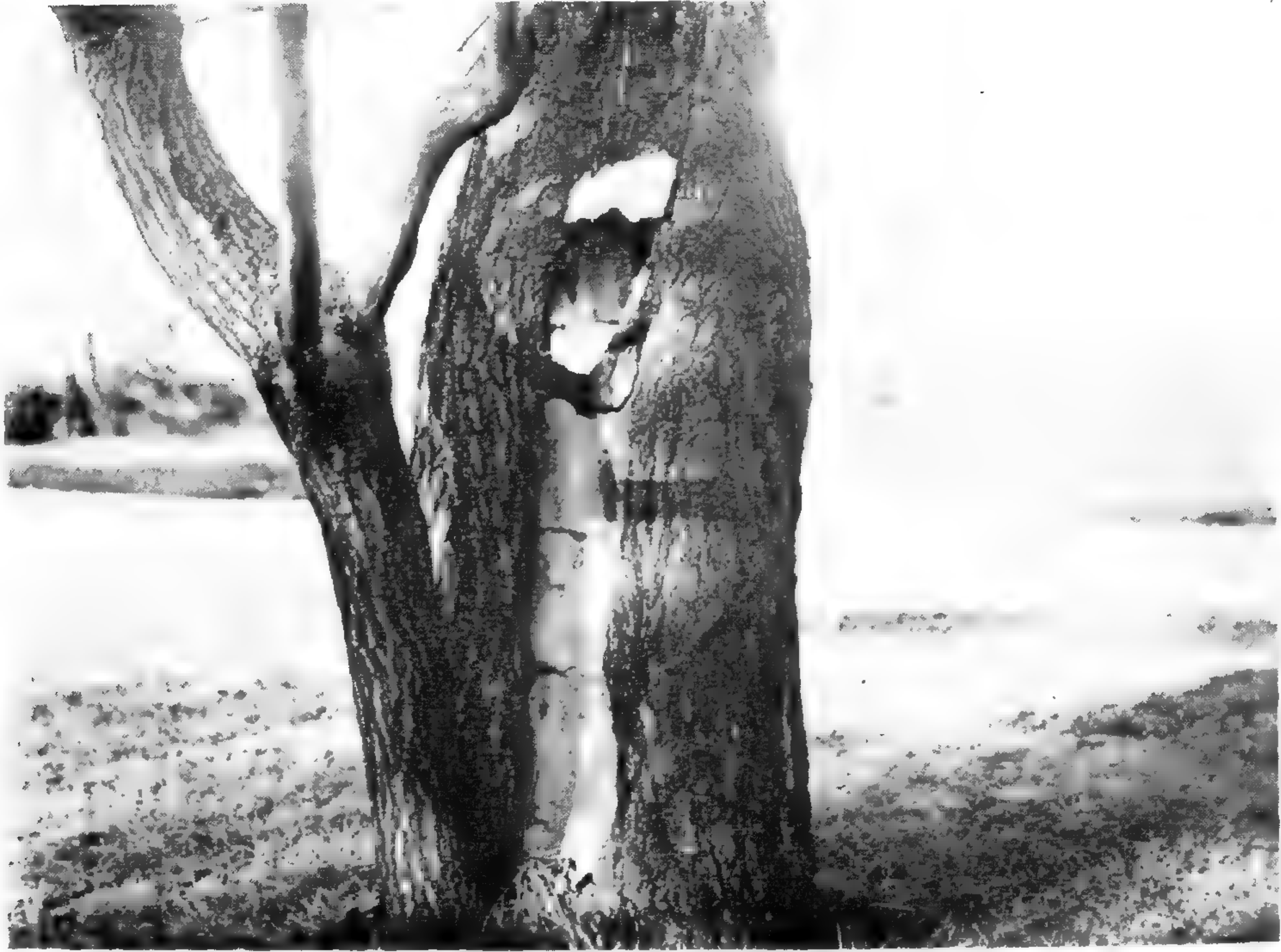
TREE IMPROPERLY FILLED WITH CONCRETE.
