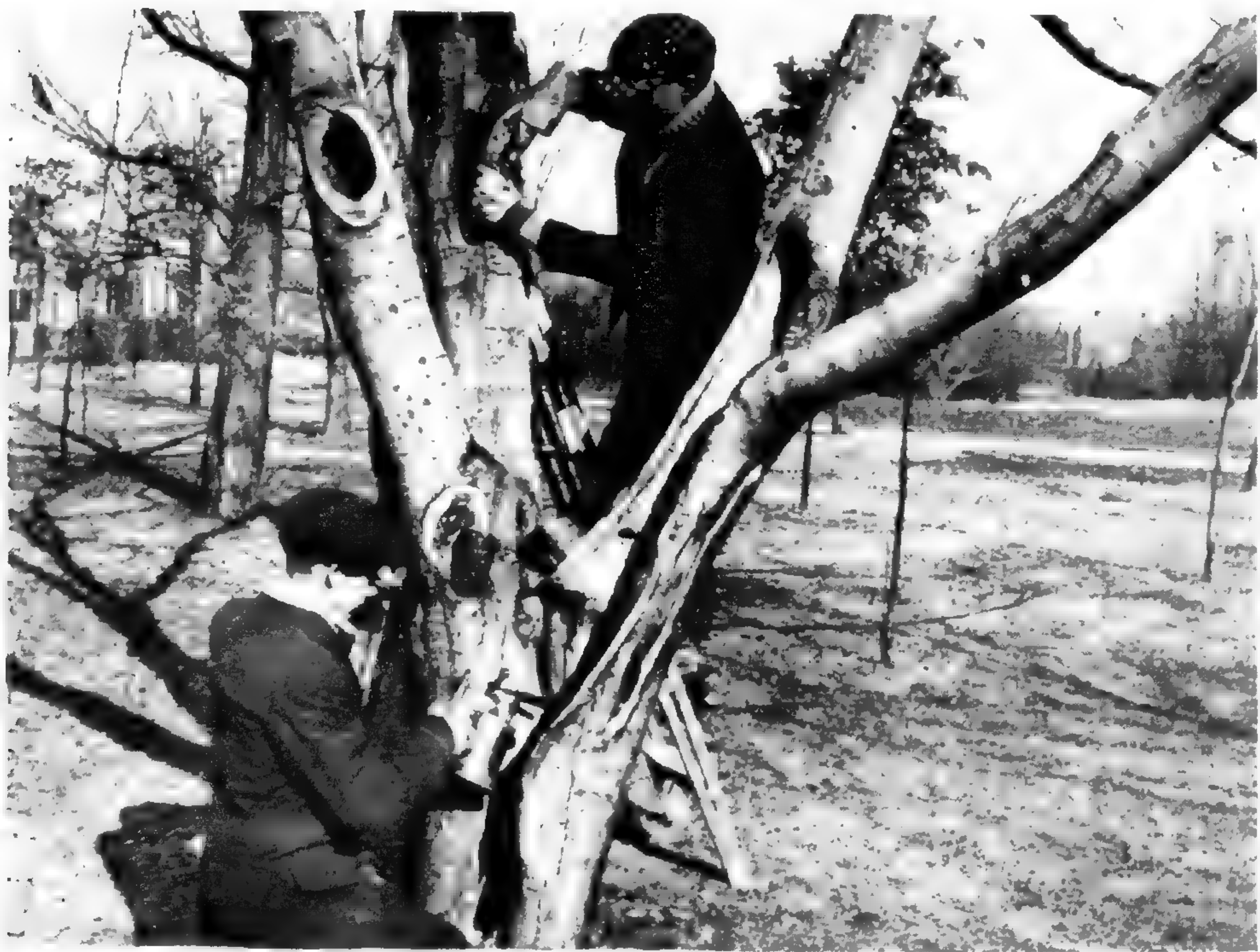
EXCAVATING AND BURNING OUT WITH TORCH.
