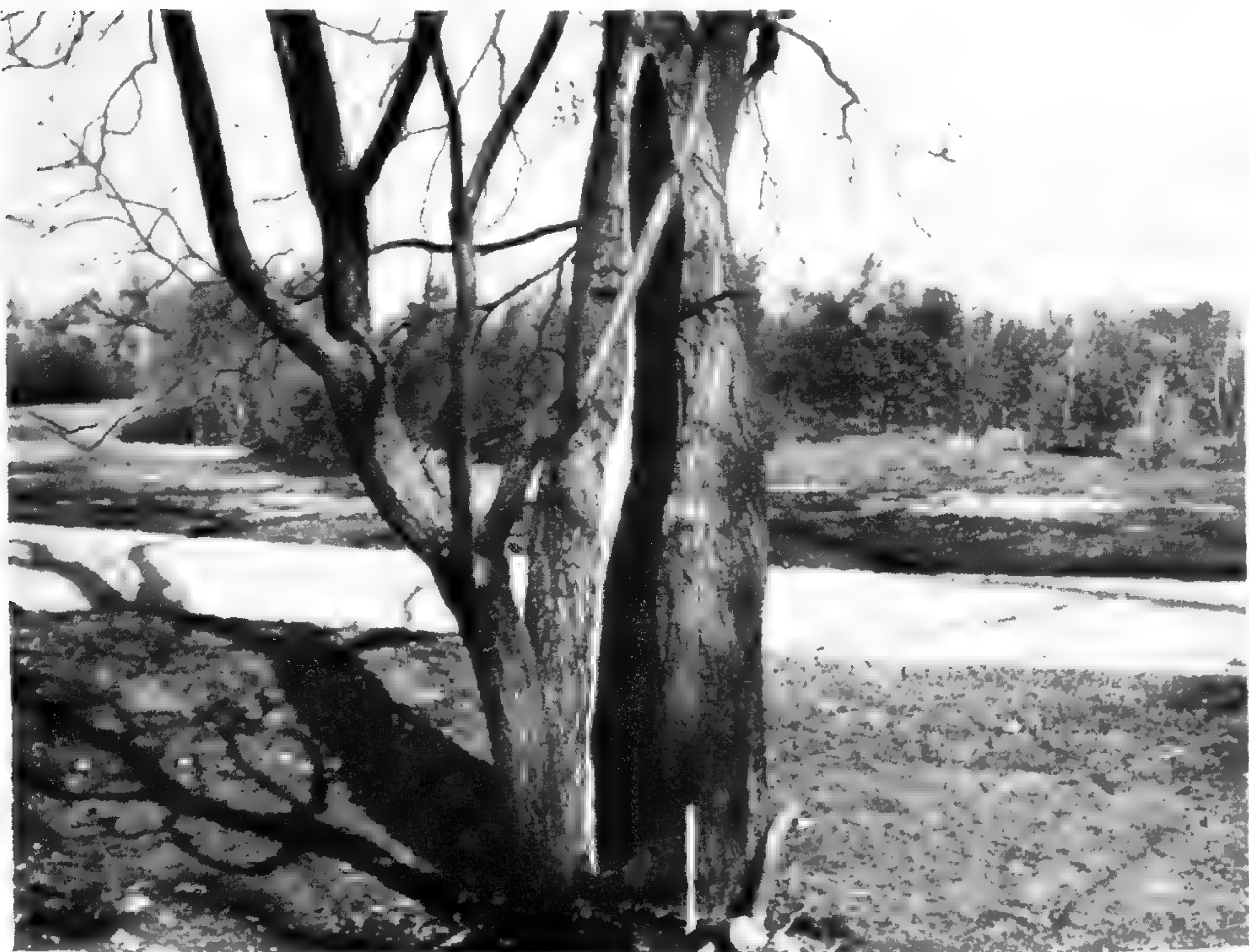
OLD FILLING TAKEN OUT AND CAVITY EXCAVATED.
