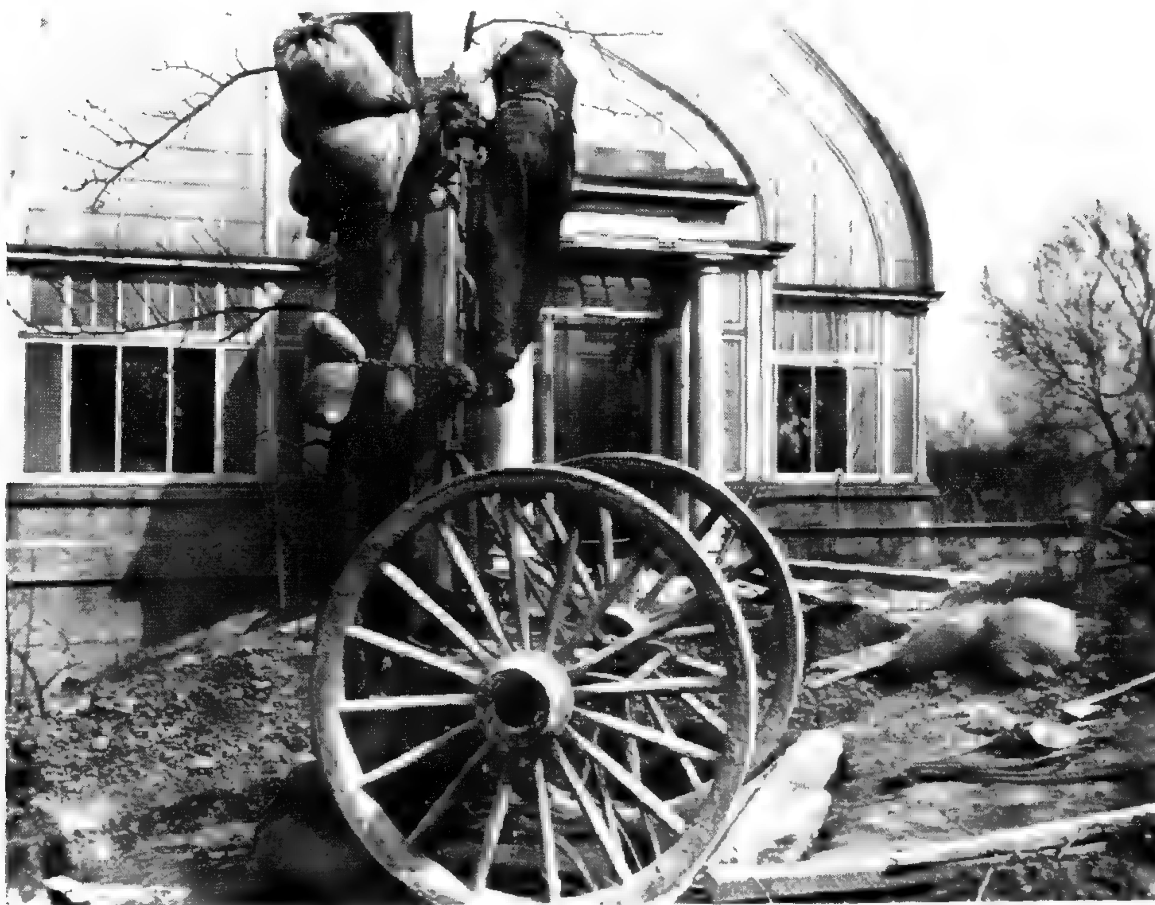
ATTACHING THE BOOM TO THE TRUNK OF THE TREE.
