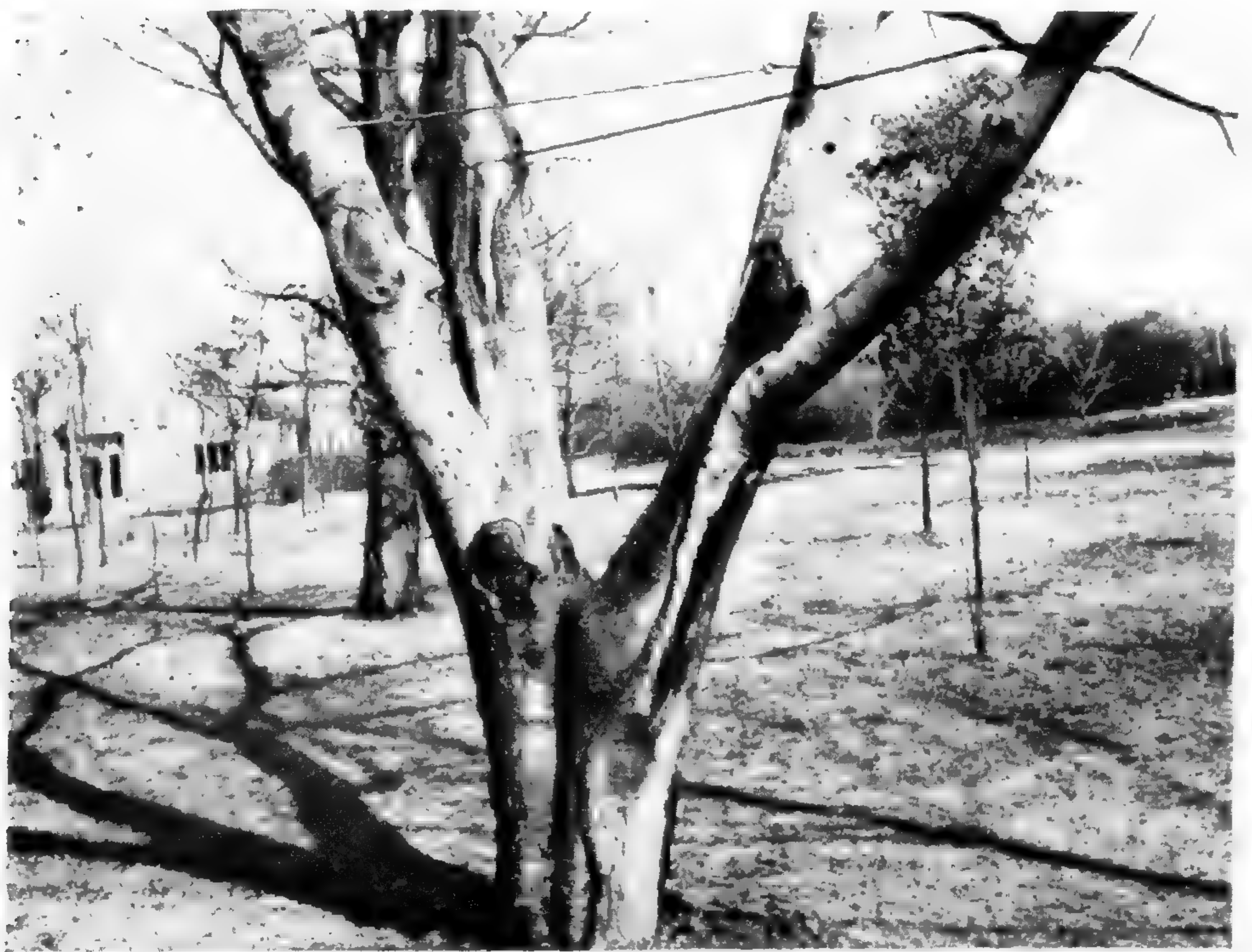
FILLED WITH CONCRETE AND PAINTED.
