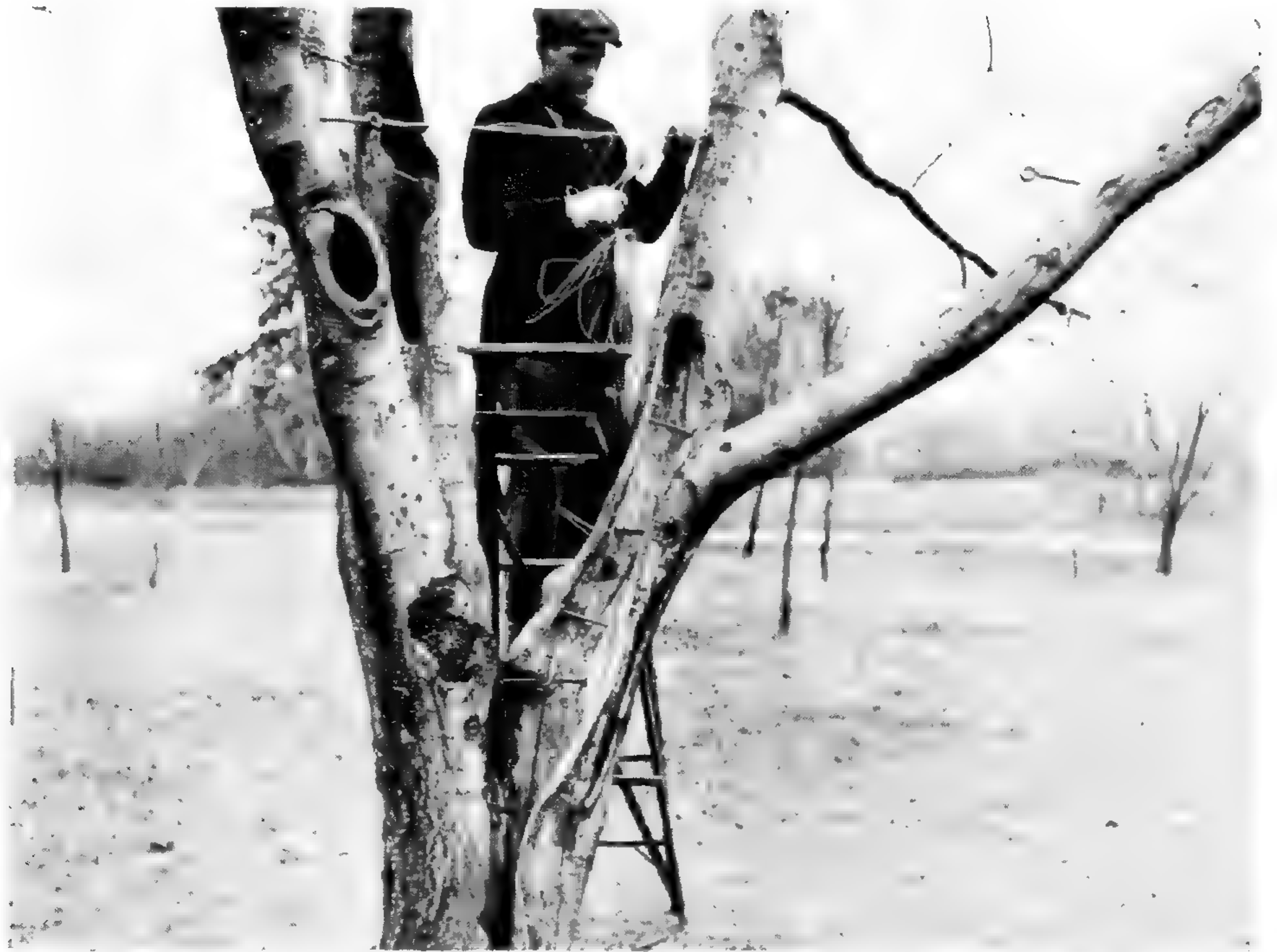
BOLTED AND BRACED.
