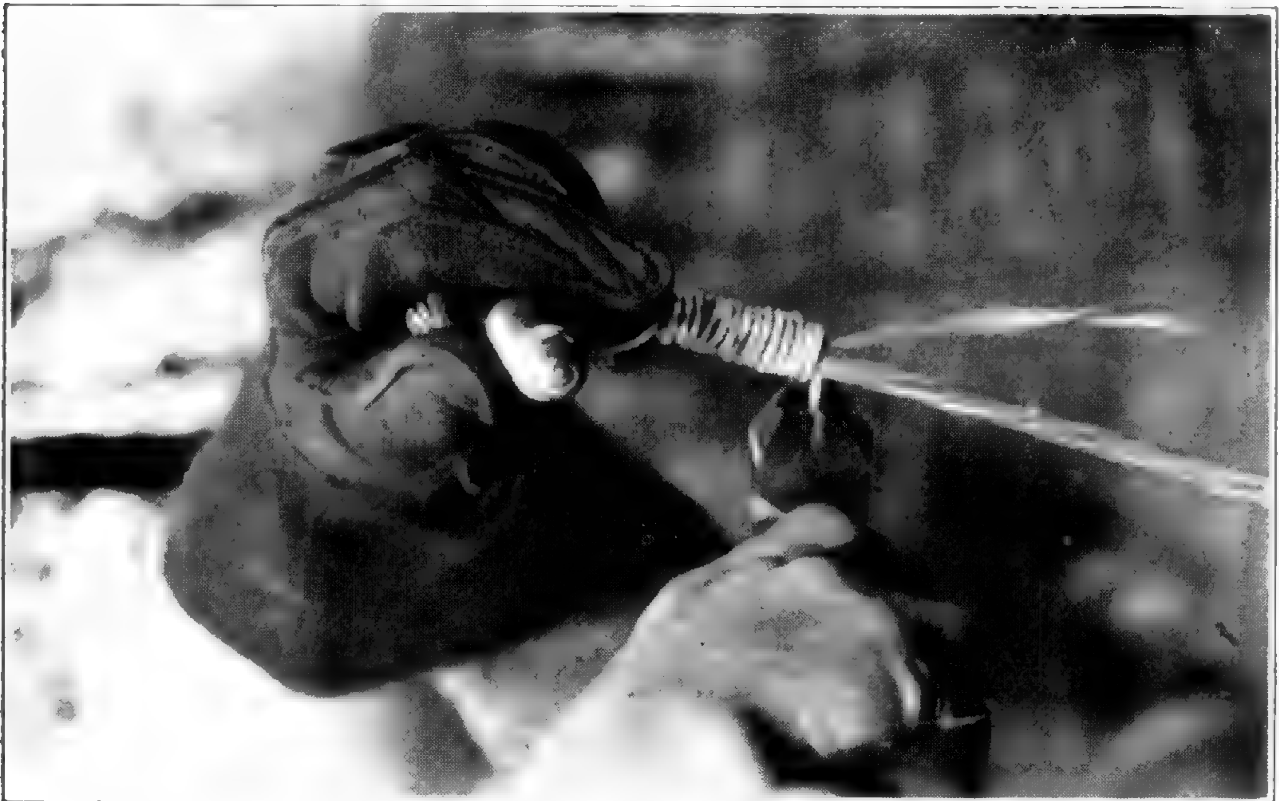
METHOD OF WRAPPING CABLE.
