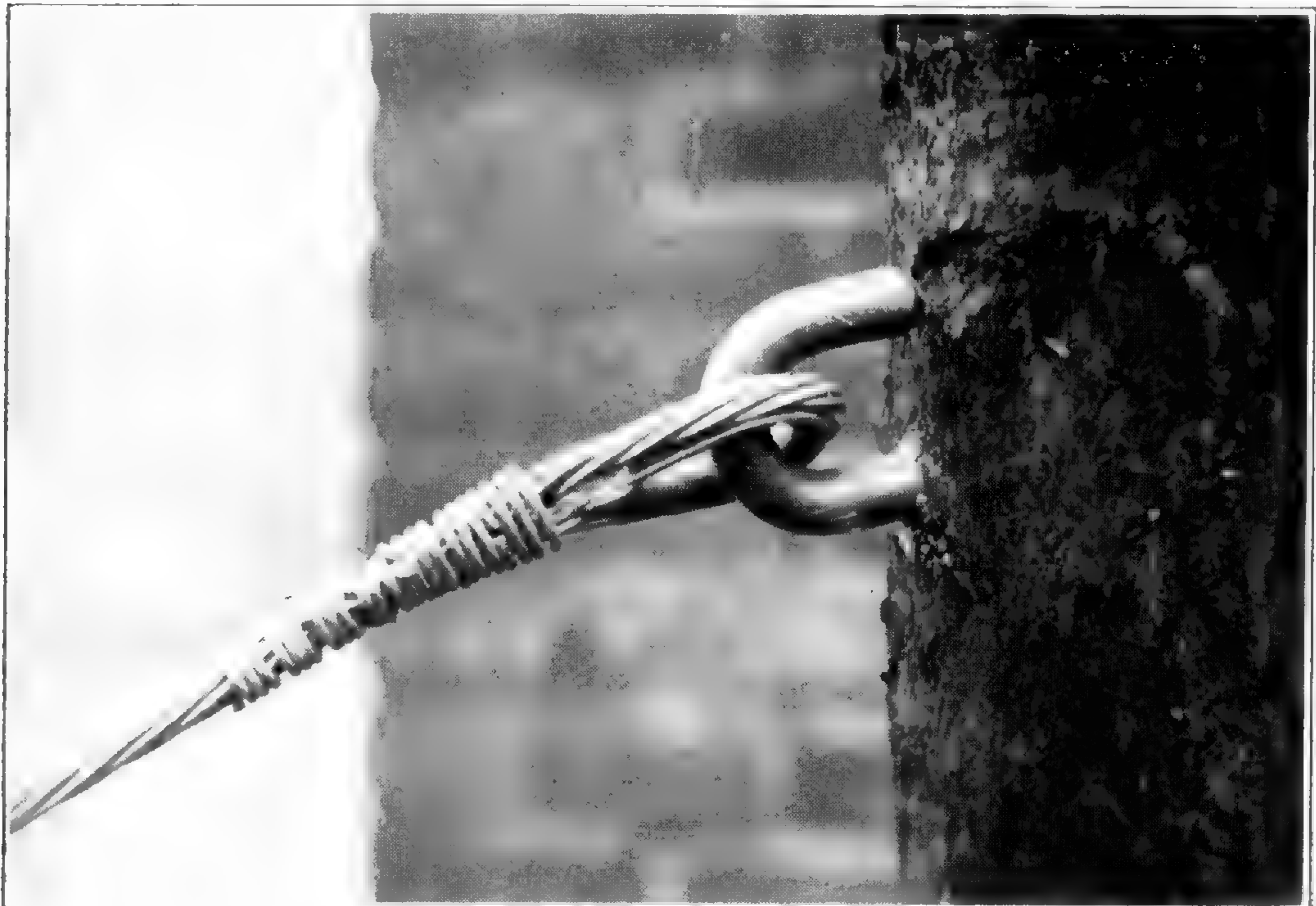
CABLE AFTER INSTALLATION, SHOWING LAG HOOK TURNED UP.
