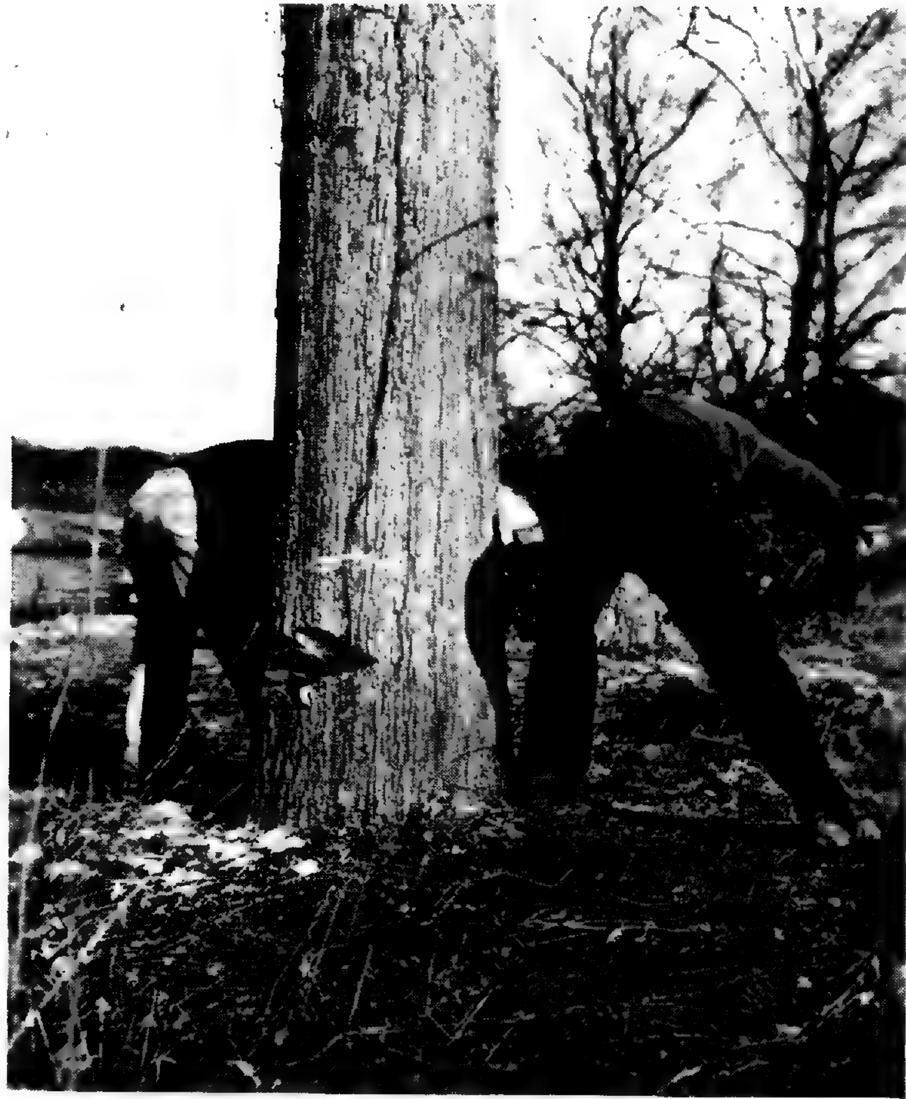
Showing the notch and the use of the cross-cut saw
