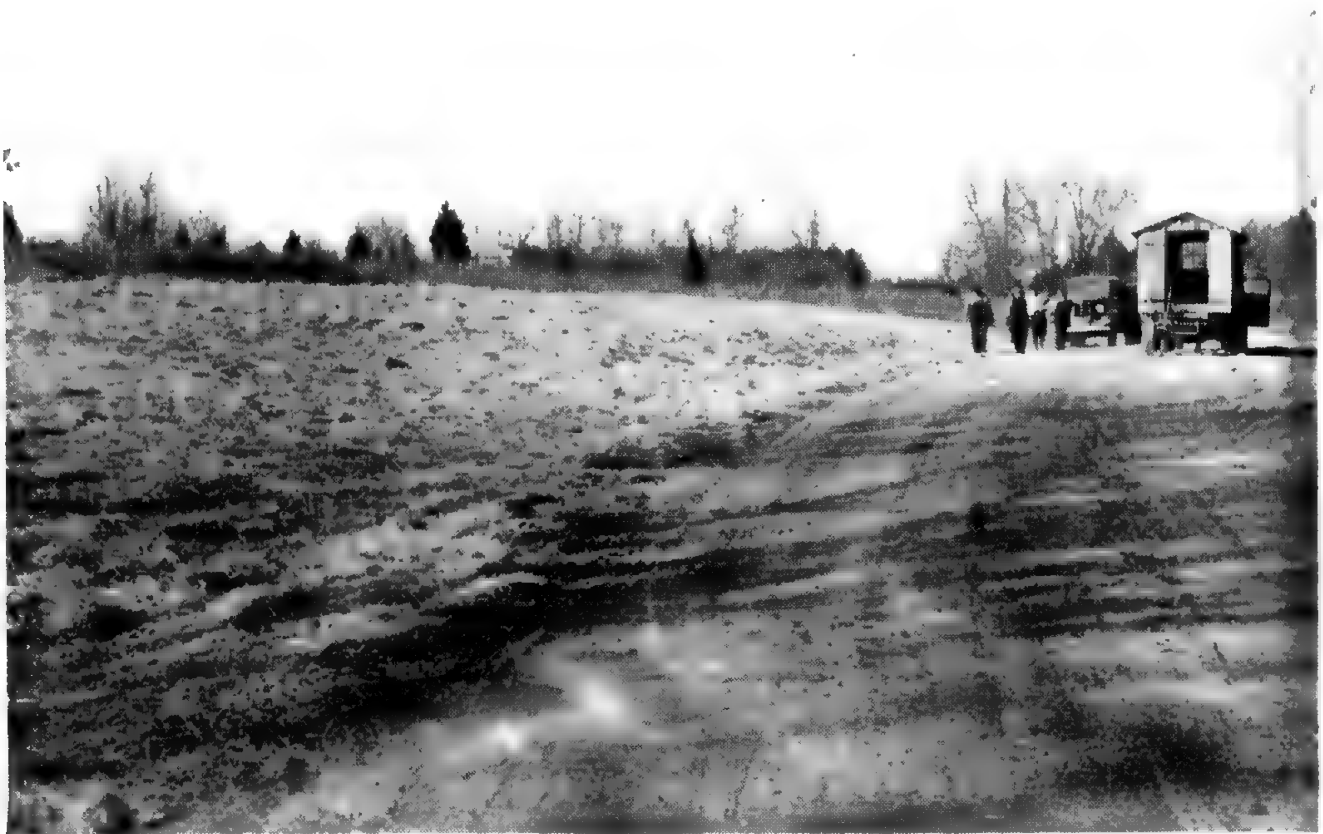
Grading finished and shoulders mulched with straw
