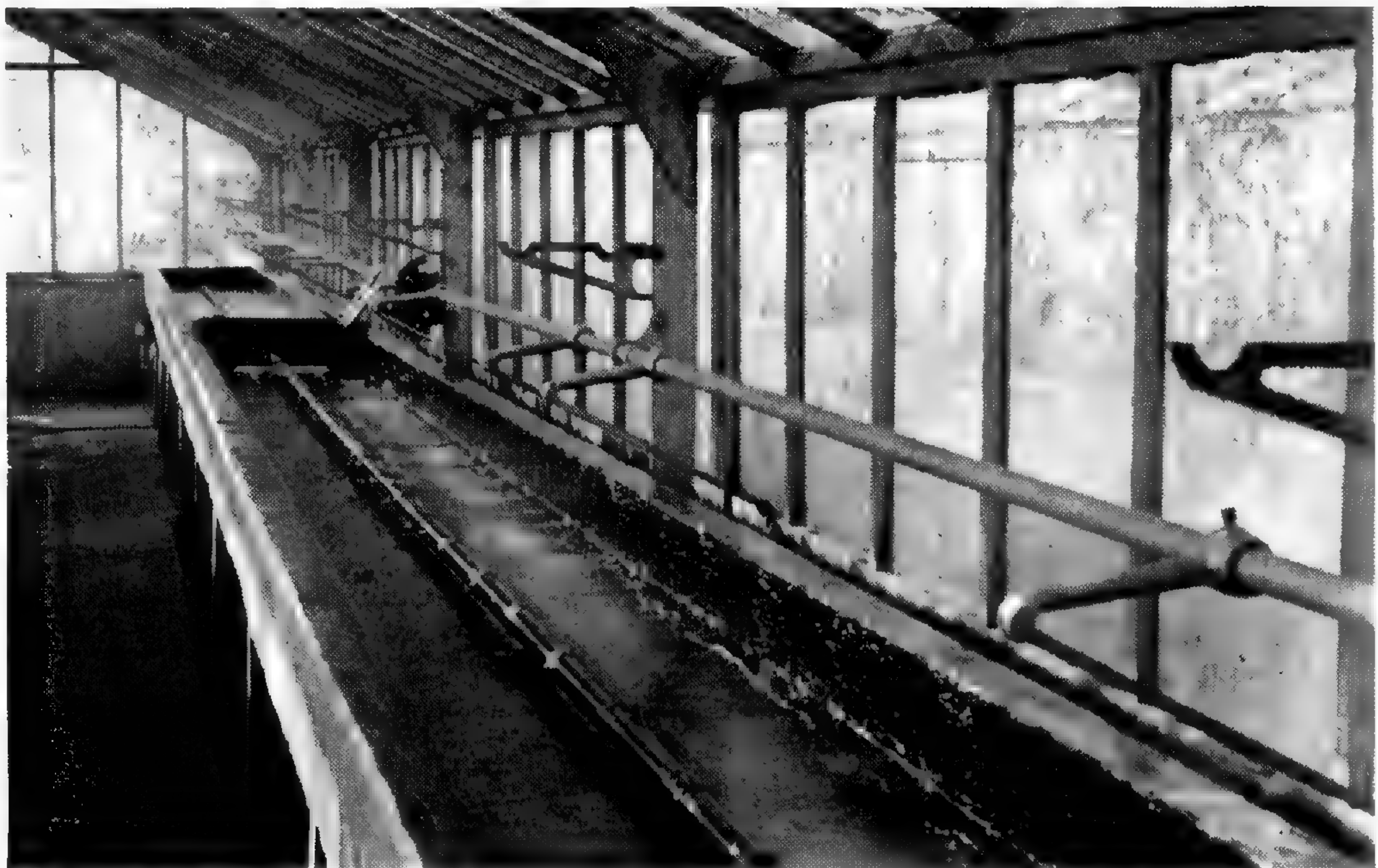
Hydroponics bench painted and ready for gravel. Note intake box with perforated pipes extending to ends of bench for rapid distribution of the nutrient solution.
