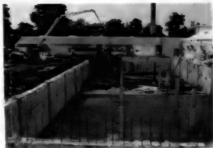
Workmen preparing new foundation
