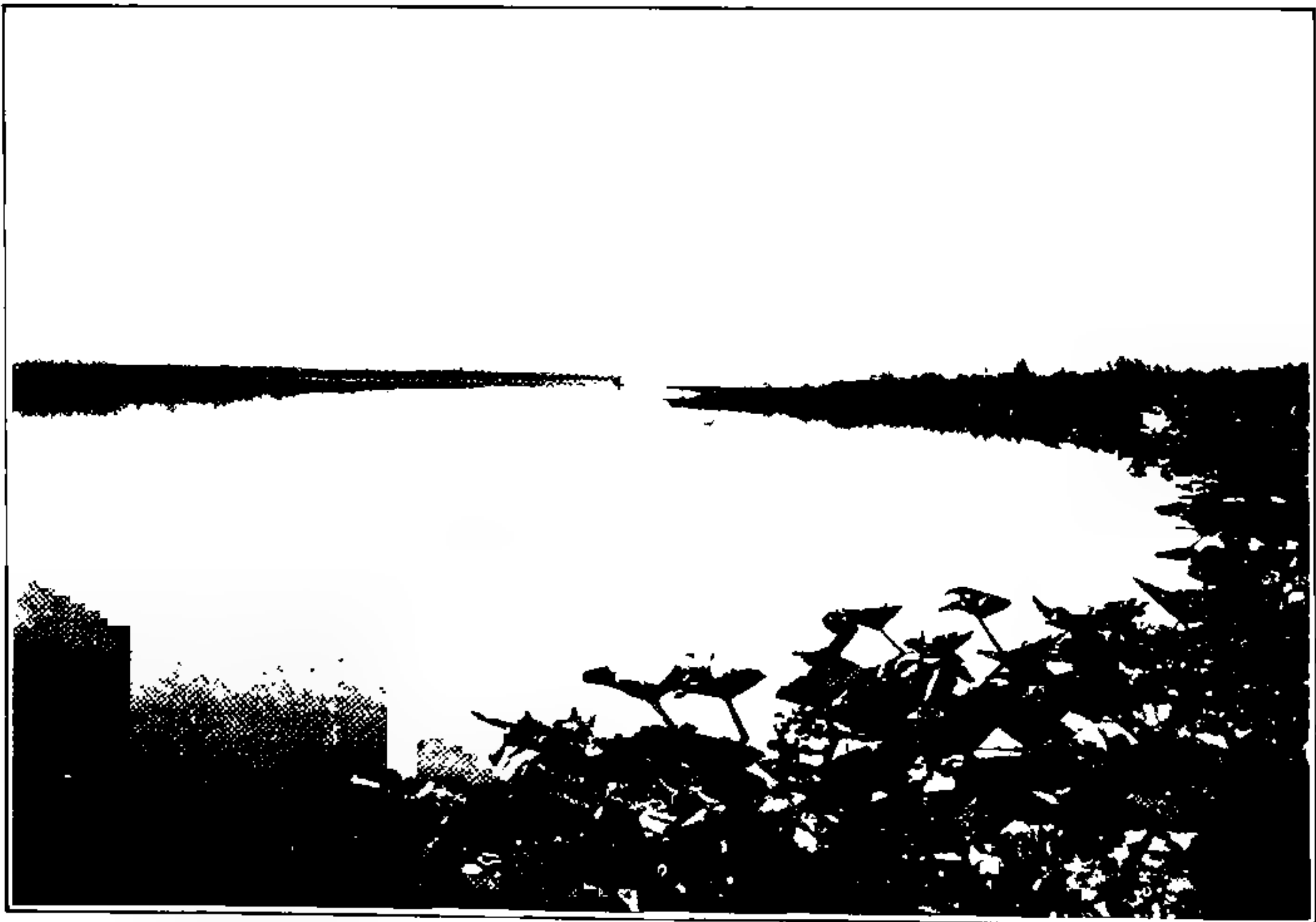
Bay at the southeastern end of Lake Okeechobee. Spatter-dock or yellow pond-lily and other water-plants in the foreground. Everglades in the distance.
