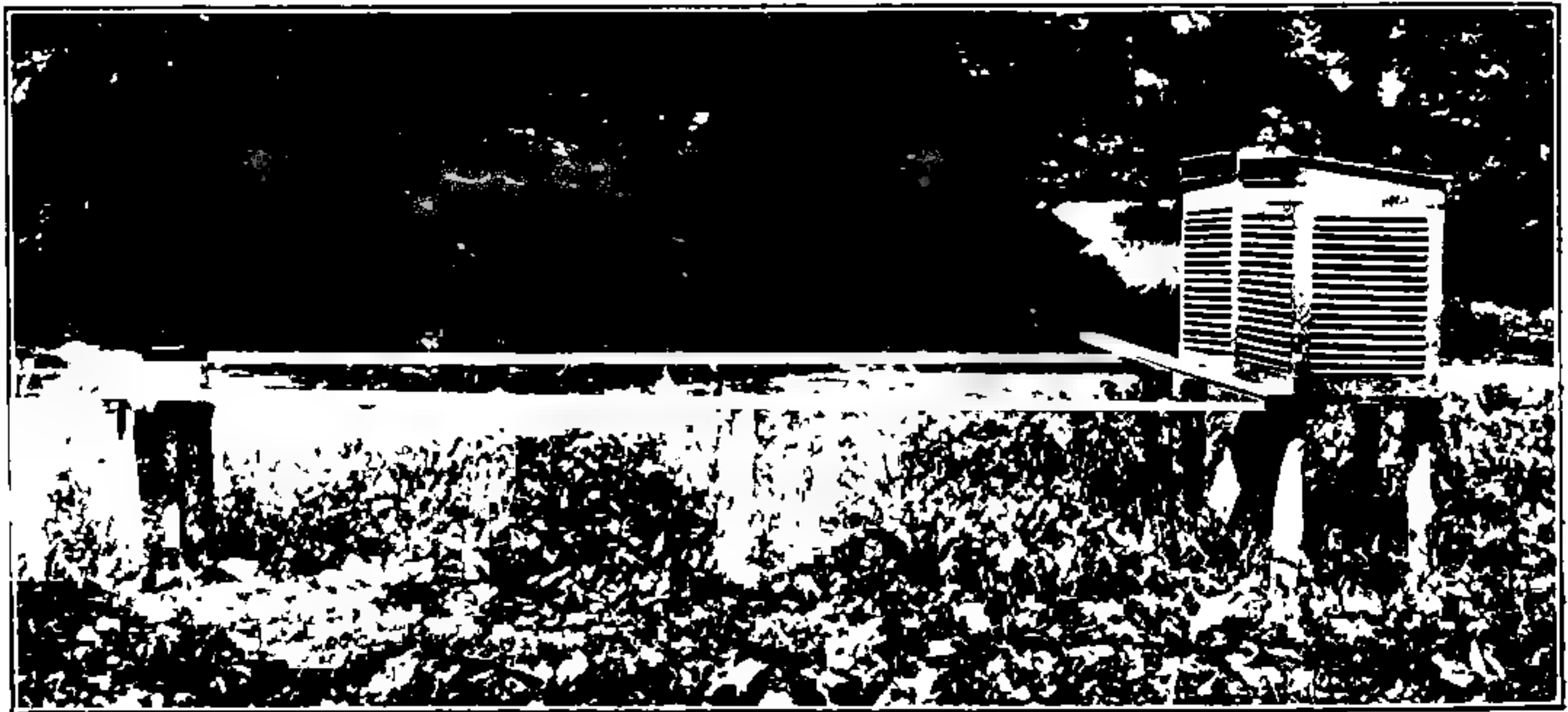
FIG. 20. Meteorological station in Garden. Rain-gauge in corner of enclosure. The bulb of the Hallock thermograph is buried in the middle of the enclosure at a depth of 30 cm. The instrument shelter at the right contains the recording and registering apparatus.
