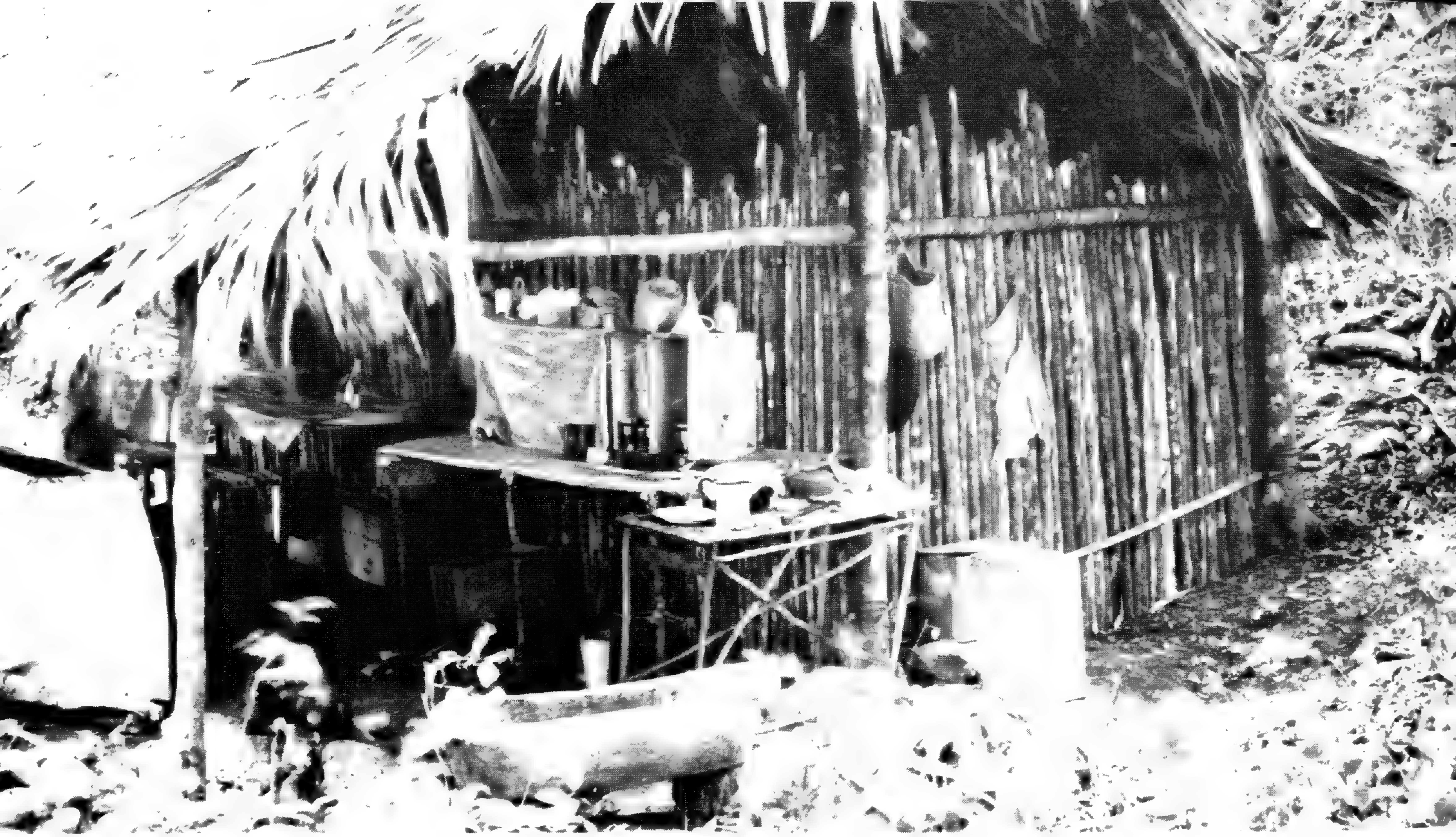
Fig. 54. Our "home" at Coba, erected in three days by two of our field men helped by two Maya Indians from Dzitnup. Built entirely of materials from the forest covering the ruins, this pole and log shelter, tied together with stems of vines and strips of bark, was thatched with leaves of the botan palm, a species of Sabal . The pole enclosed room of the house was our tarpaulin-covered floor sleeping quarters. The open side contained kitchen facilities, table, and workbench together with plant driers.
